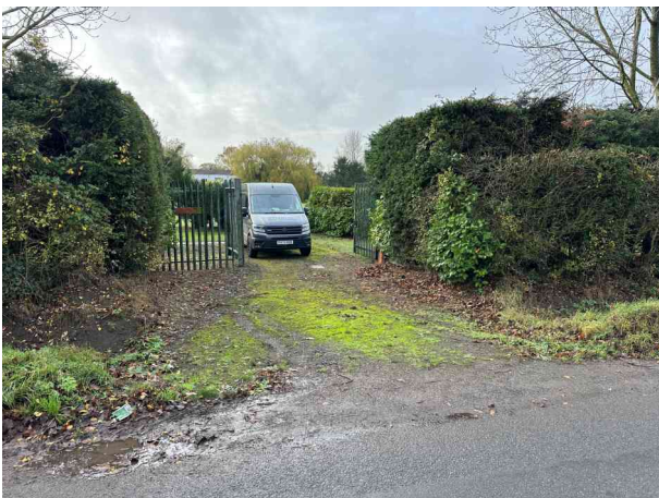
Crossover 1, no culvert
