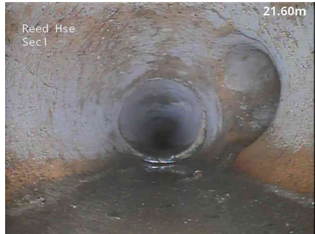
20, 00:11:51, 21.70 m Junction at 3 o'clock, 100mm dia
