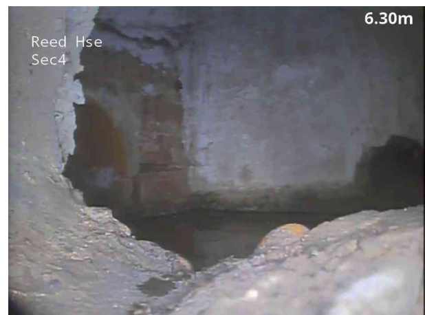
4, 00:00:36, 6.30 m Finish node, catchpit, reference: CP2, Buried, unable to access
