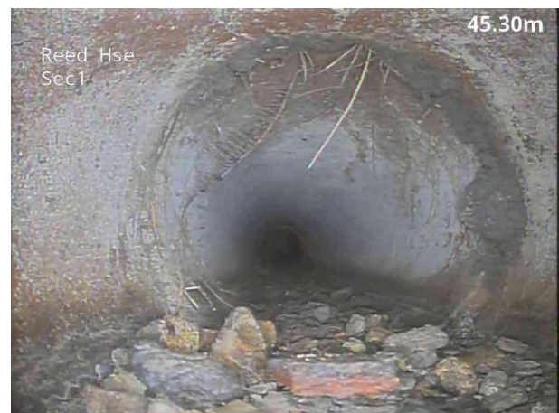
36, 00:09:06, 45.30 m Roots, fine at joint
