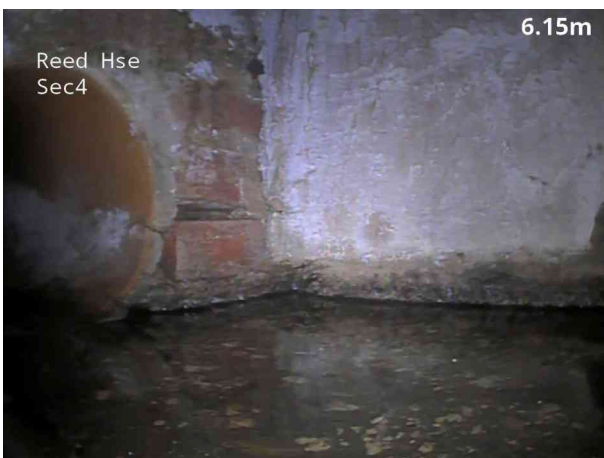
3, 00:00:36, 6.30 m Finish node, catchpit, reference: CP2, Buried, unable to access
