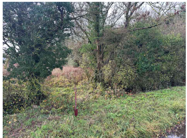
Crossover 2, no culvert
