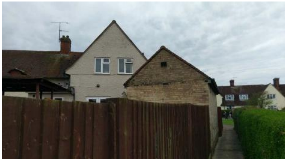
Rear view from the pedestrian side access path
