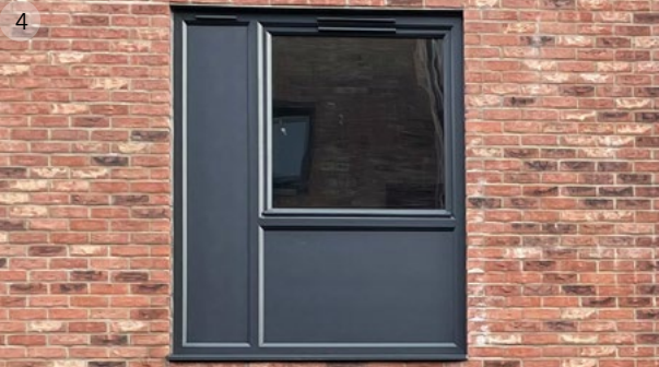
Spandrel panel to full height windows, in matching grey
