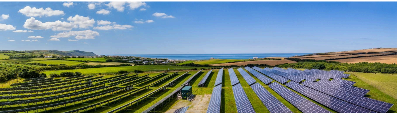
Construction Environment Management Plan – Tophams Solar
