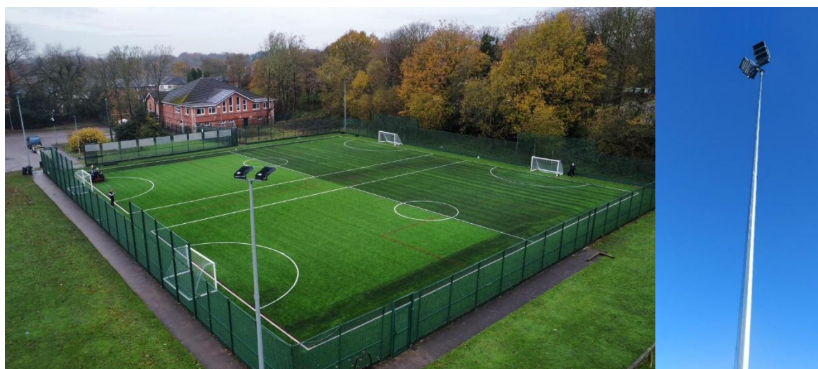
Figure 3 - Example of 11m High Slimline Floodlighting Column With LEDs
