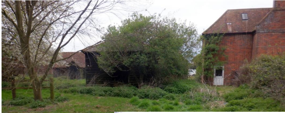
Rear Elevation prior to implementation of permissions 23/00559/LBC and 23/00558/FPH
