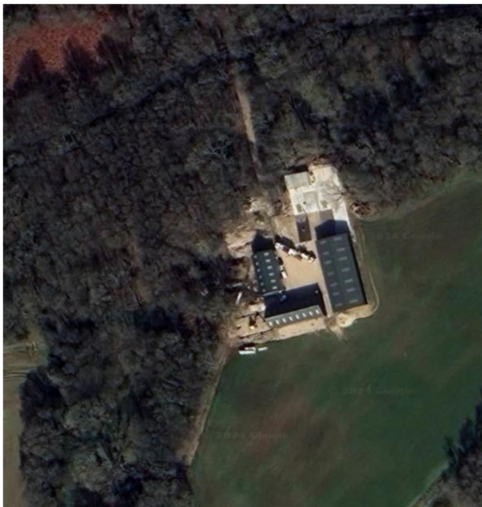
Figure 2: Aerial image of the application site.
