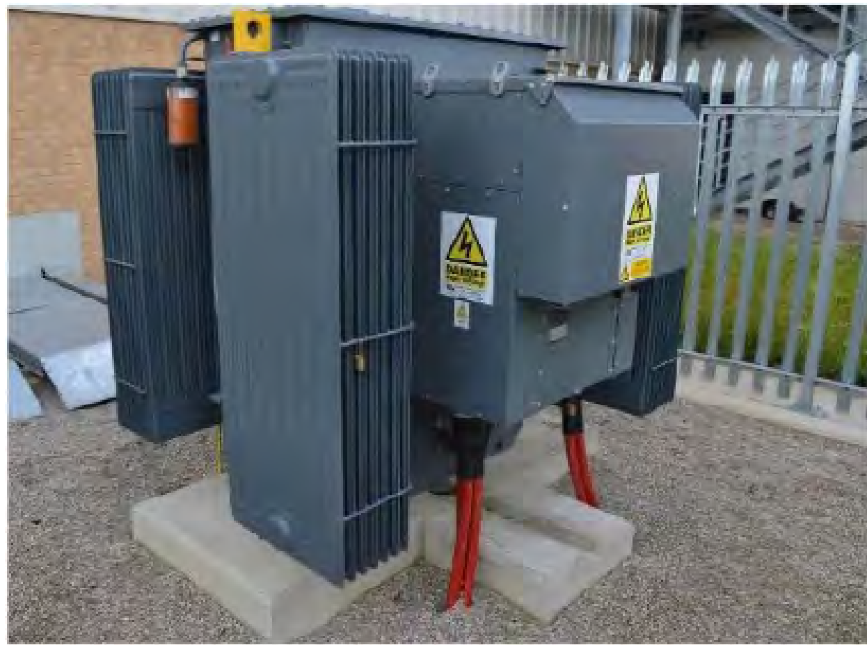
Left and middle: Outdoor package substation, fenced without enclosure Right: 1500kVA pre-fabricated MDS for electric vehicle charging application
