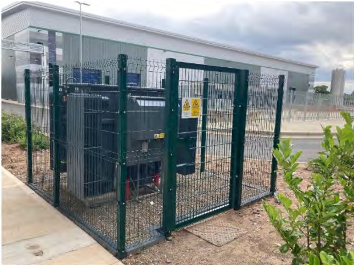
Left and middle: Outdoor package substation, fenced without enclosure Right: 1500kVA pre-fabricated MDS for electric vehicle charging application
