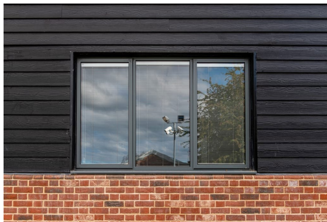
UPVC flush casements windows. Double glazed. Frame Colour: Black
