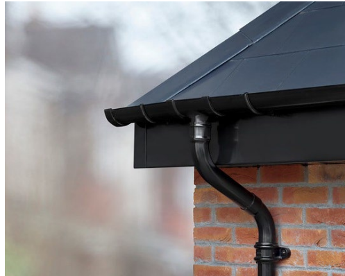
Treated timber painted black soffit and fascia board
