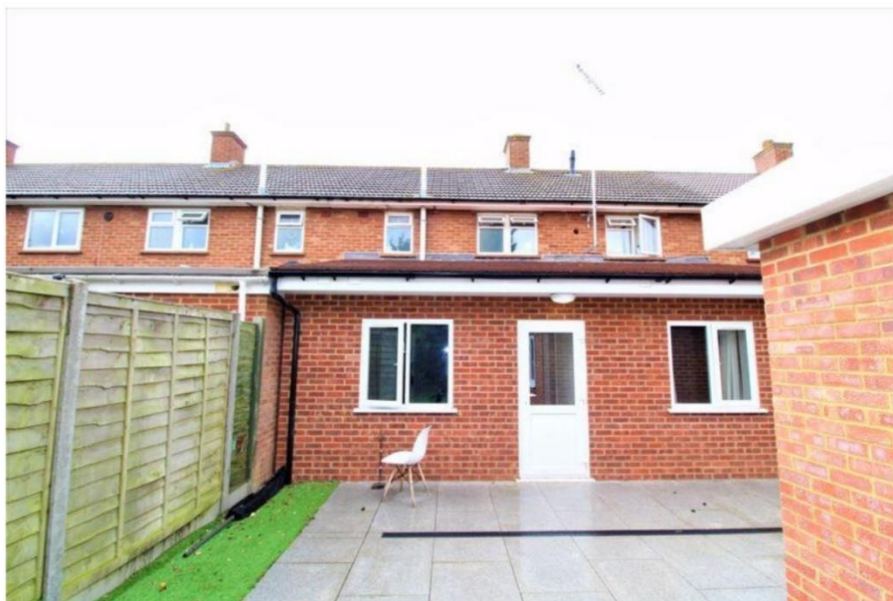
Figure I: Photograph of the property
