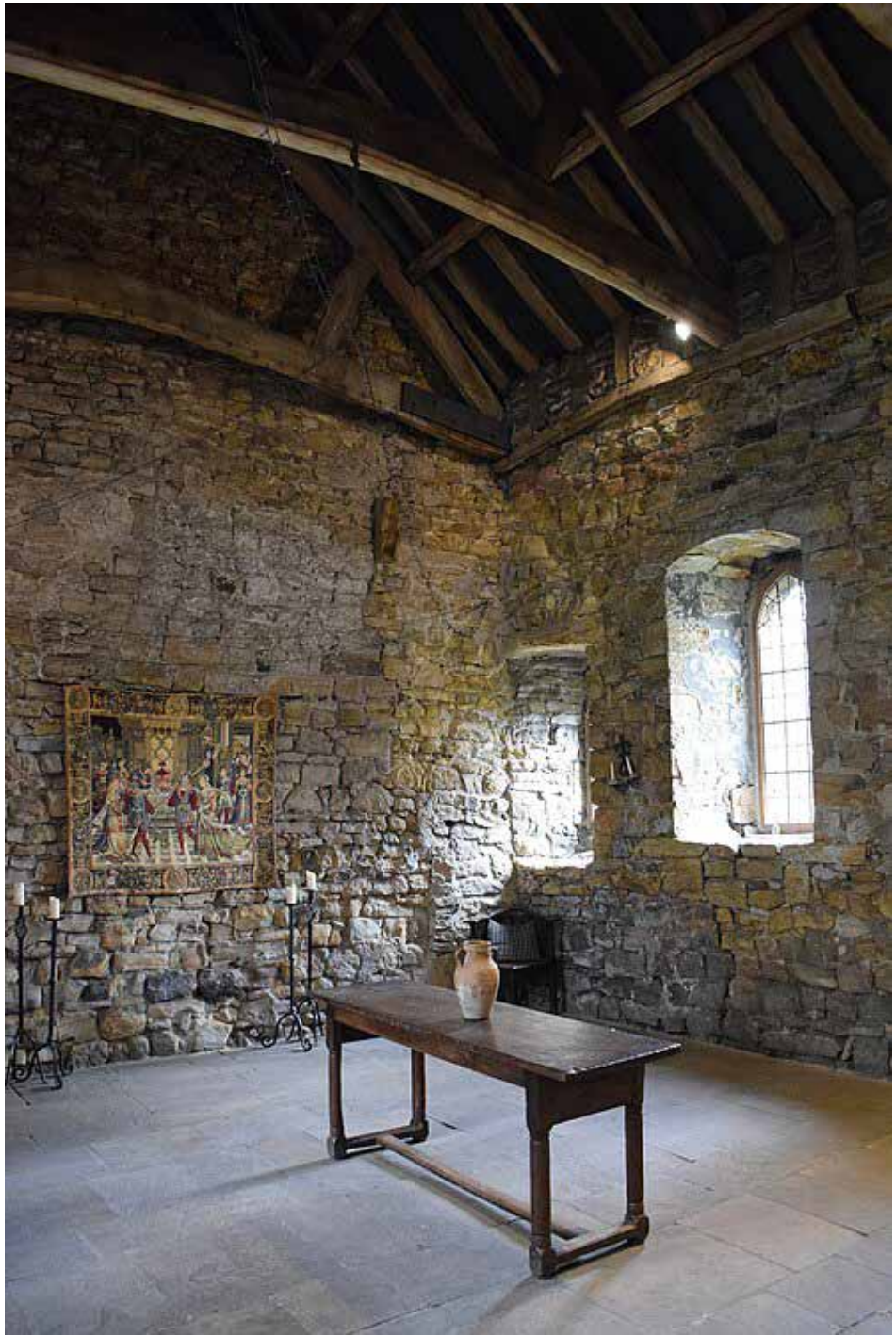
14th century open hall at Crook Hall, Durham
