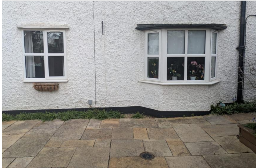
EXISTING (SSE) Side
