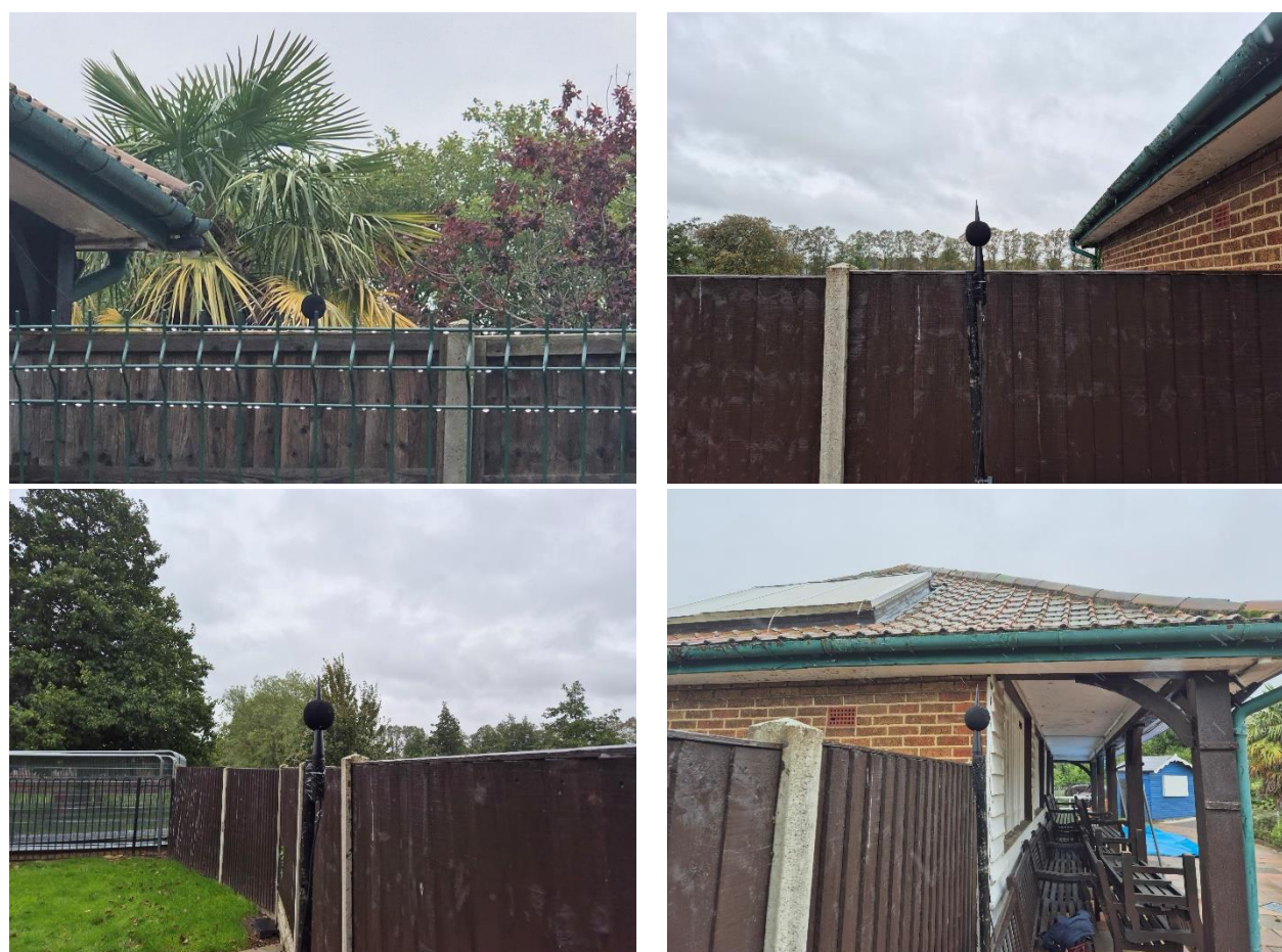
Figure A.2.2 Fixed measurement F1 location in situ
