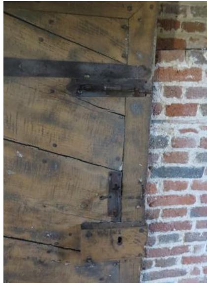
Figure 4.90: Showing an historic bolt and Suffolk latch on the dining room side of the 3-plank door.
