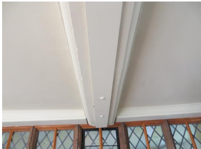
Figure 4.99: Showing one ovolo moulded ceiling beam.
