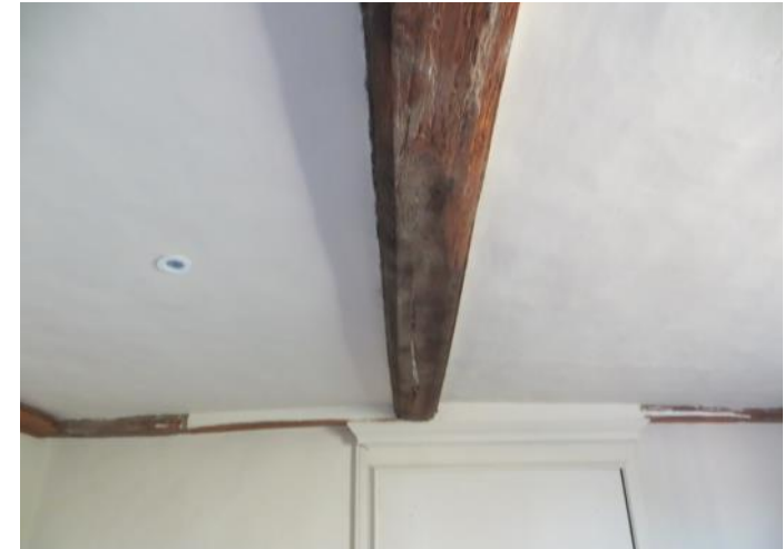
Figure 4.151: Showing an historic ceiling beam in the room.
