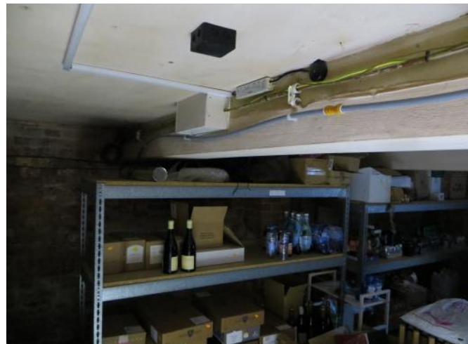
Figure 4.111: Showing the concrete beam in the cellar.
