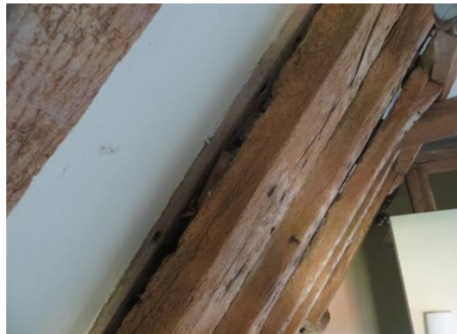
Figure 4.188: Showing some partnered rafters in the south-eastern bedroom at loft level.
