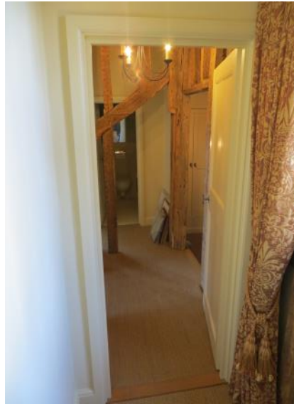
Figure 4.146: Showing the 2-panelled door and doorway adjoining the 17th century 4-light window.
