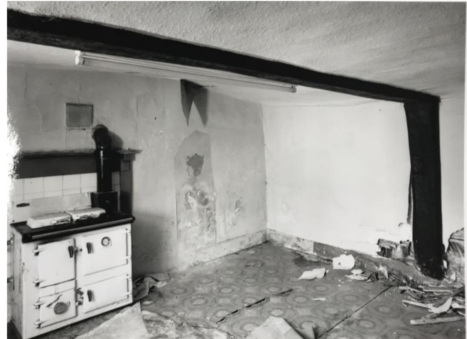
Figure 4.18: 1992-94 photograph showing the kitchen on the ground floor of the kitchen cross wing (Source: Historic England Archives).
