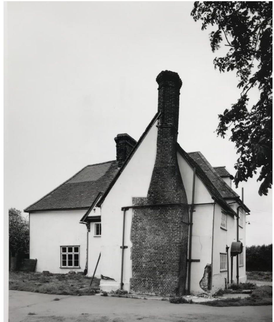
Figure 4.6: 1992-94 photograph (Source: Historic England Archives). Showing the southern elevation of the kitchen cross wing.
