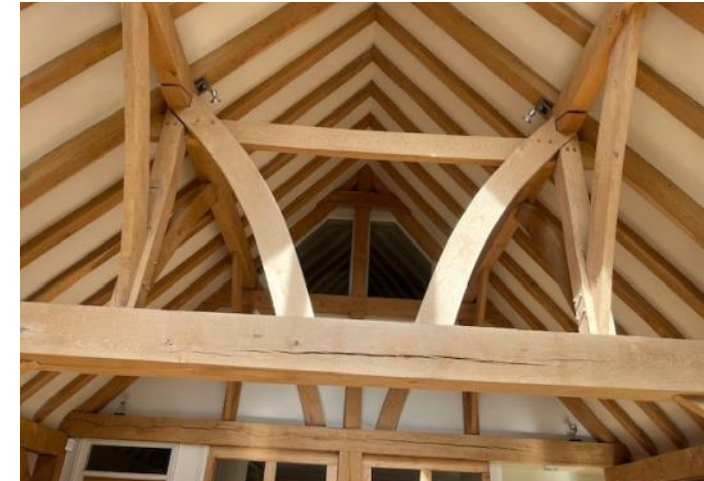
Figure 4.124: Showing a typical purlin roof truss within the interior of the garden room.
