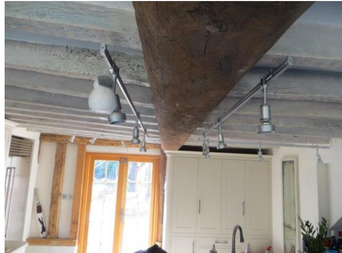
Figure 4.120: Showing the chamfered beam in the kitchen.
