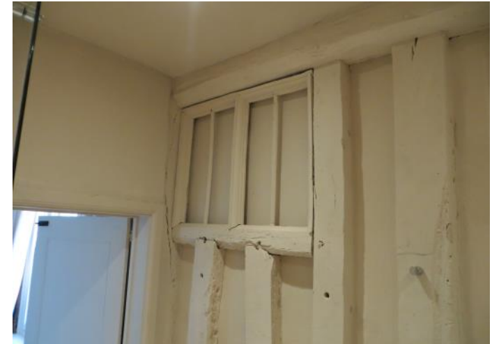
Figure 4.158: Showing northern wall of the north-eastern shower room. Note the former window (part).
