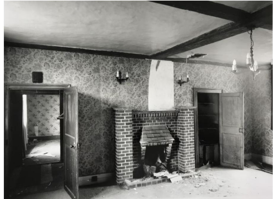
Figure 4.12: 1992-94 photograph showing the ground floor western room in the main range (sitting room) and its fireplace (Source: Historic England Archives). Also shown is the doorway towards the entrance lobby (left) and a door into a cupboard (right).
