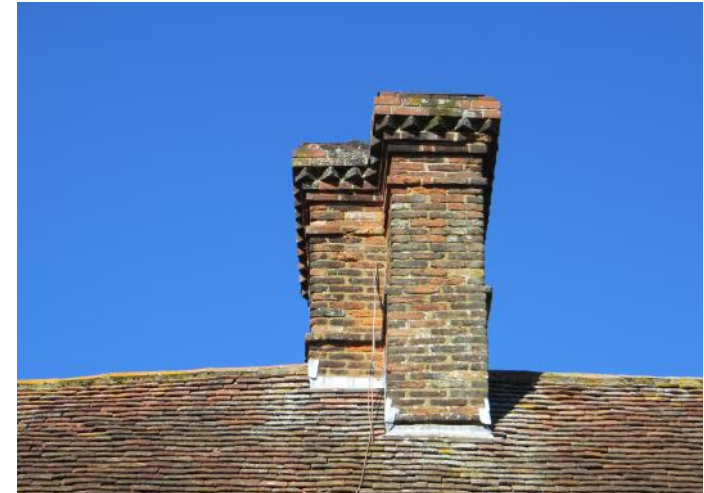
Figure 4.81: Showing the corniced stack in the centre of the main range's roof.
