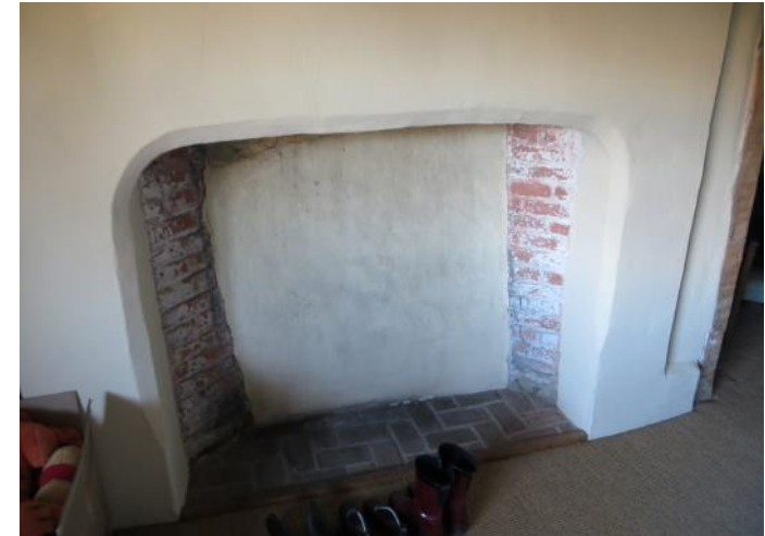
Figure 4.170: Showing the fireplace in the south-eastern bedroom.
