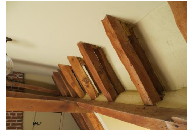
Figure 4.183: Showing partnered rafters in the south-eastern bedroom at loft level.
