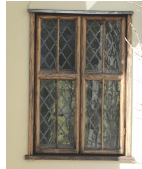
Figure 4.71: Showing the eastern ground floor window on the main range.
