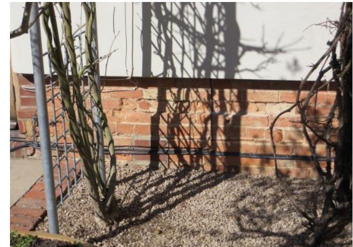
Figure 4.77: Showing the plinth brickwork east of the French windows.
