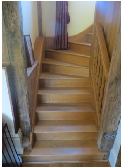
Figure 4.127: Showing the stair wing as seen from the dining room.
