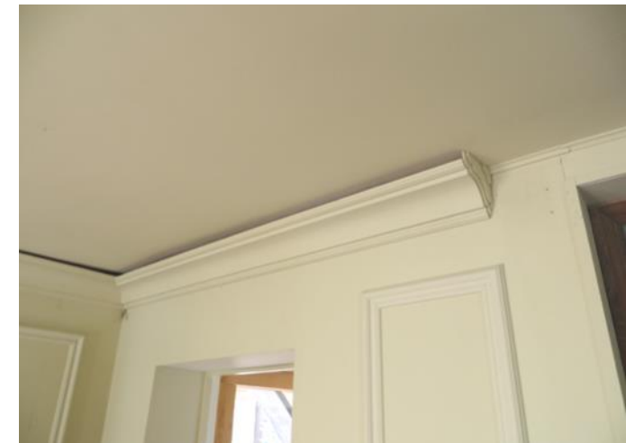
Figure 4.100: Showing a length of modern cornice.
