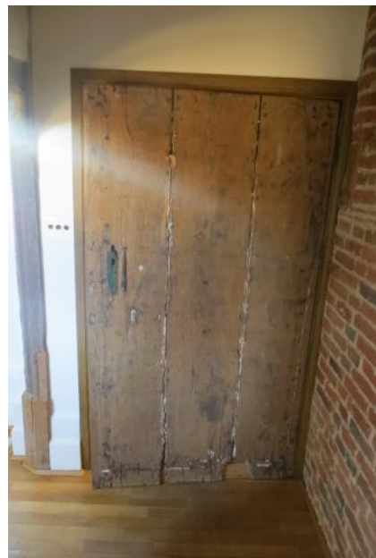
Figure 4.88: Showing the historic 3-plank door that once served the front entrance and today serves the doorway from the dining room into the lobby.
