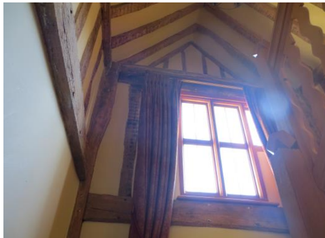
Figure 4.129: Showing the first floor level of the stair wing.
