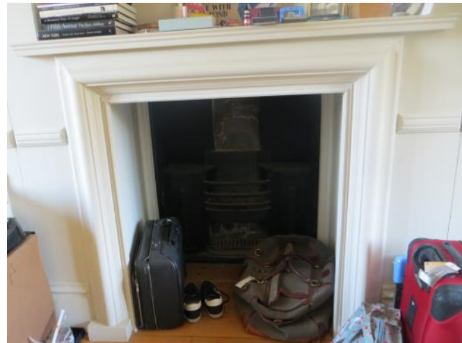
Figure 4.135: Showing the chimneypiece and hob grate.
