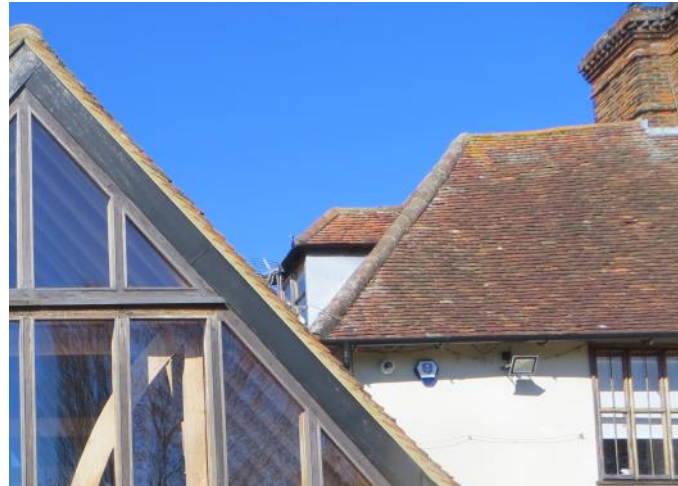
Figure 4.84: Showing the dormer on the main range's western roofslope.
