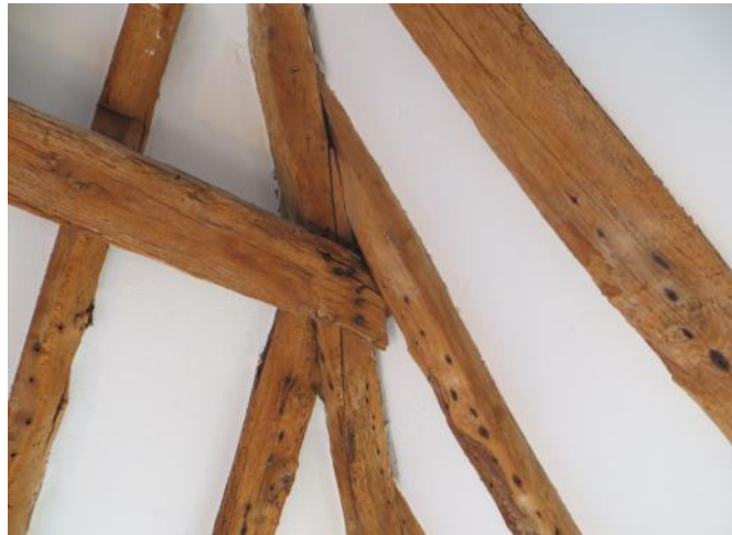
Figure 4.192: Showing clout nailed timbers in the western bedroom's roof at loft level.
