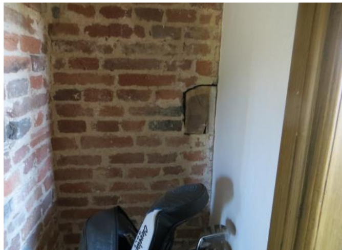
Figure 4.92: Showing the sitting room fireplace's bressummer as seen from the lobby.
