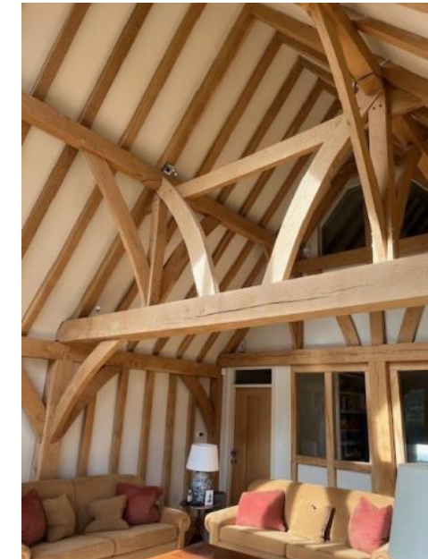
Figure 4.124: Showing a typical purlin roof truss within the interior of the garden room.
