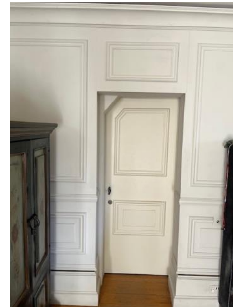
Figure 4.134: Showing the doorway from the western bedroom into the bathroom at first floor level within the garden room.
