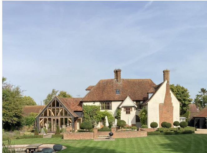
Figure 4.64: Showing the southern elevation.
