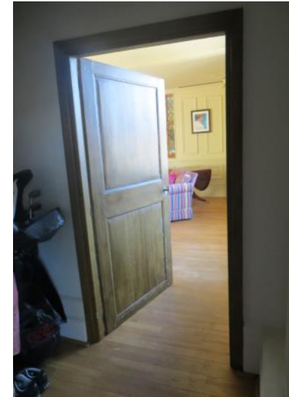
Figure 4.91: Showing the doorway from the lobby into the sitting room.
