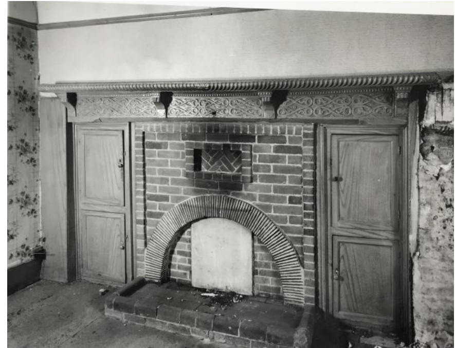
Figure 4.10: 1992-94 photograph showing the interior of the ground floor eastern central room (dining room) looking south-west (Source: Historic England Archives, Reference: BB92/06142).
