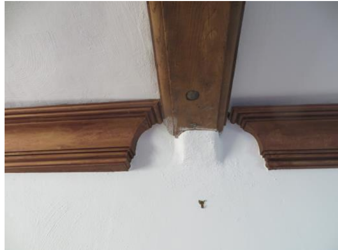
Figure 4.105: Showing the trimmed fireplace arch above the dining room fireplace.
