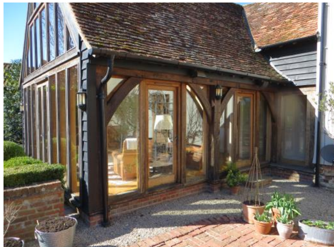
Figure 4.82: Showing the eastern return elevation of the garden room.
