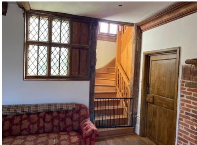
Figure 4.103: Showing the dining room doorway leading to the stair wing. Also showing the historic 3-light window, with one light blocked by the stair wing.
