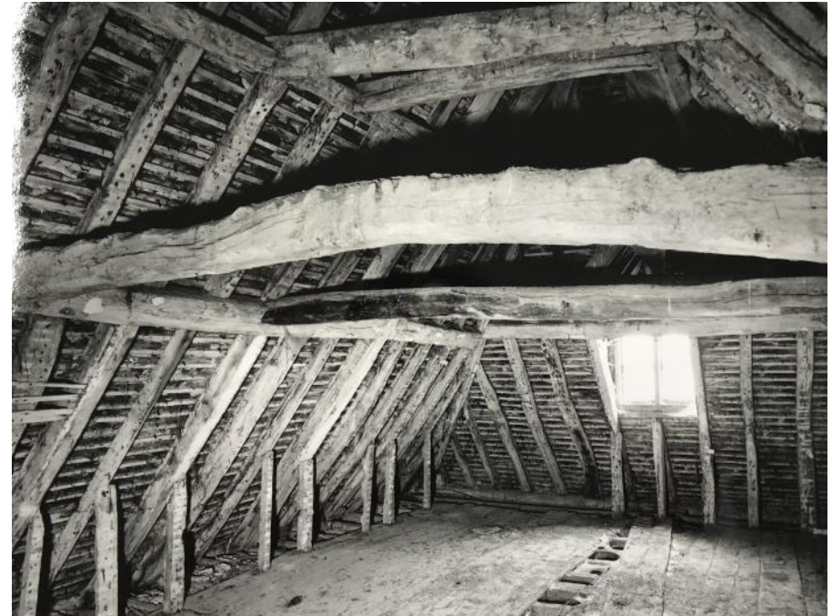
Figure 4.22: 1992-94 photograph showing the interior of the roof space of the main range (Source: Historic England Archives, Reference: BB92/06155). Figure 4.37 from 1992 confirms that the only location of a dormer window extant at that time was at the eastern end of the main range. Figure 4.22 therefore shows the area today known as the north-eastern bedroom at loft level in 1992.
