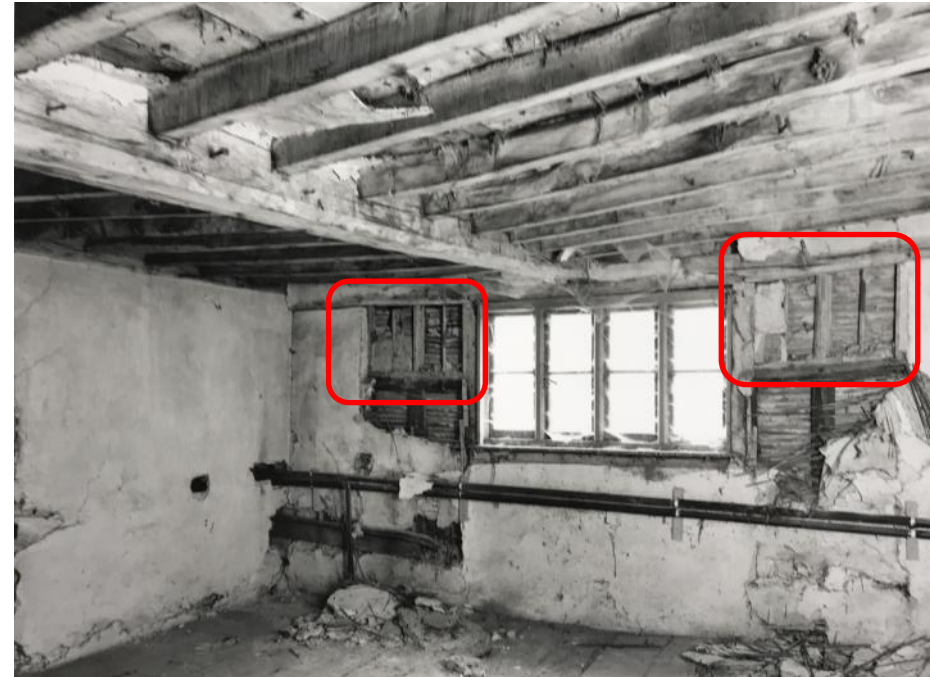
Figure 4.20: 1992-94 photograph showing the south-eastern bedroom at first floor level within the kitchen cross wing (Source: Historic England Archives). Note the upper parts of the historic windows visible to either side (marked in red).
