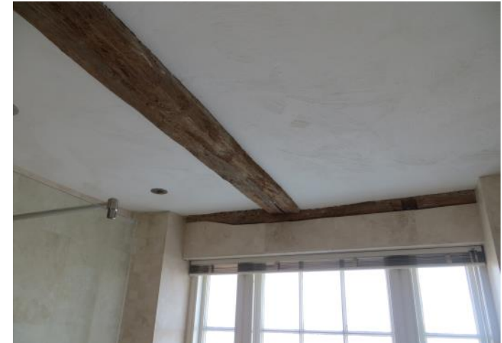
Figure 4.162: Showing historic ceiling beam and part of the wallplate in the north-eastern bathroom.
