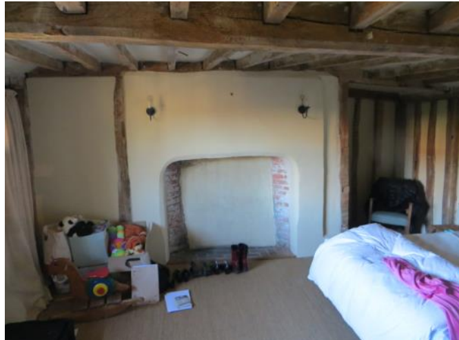
Figure 4.169: Showing the southern wall of the south-eastern bedroom.
