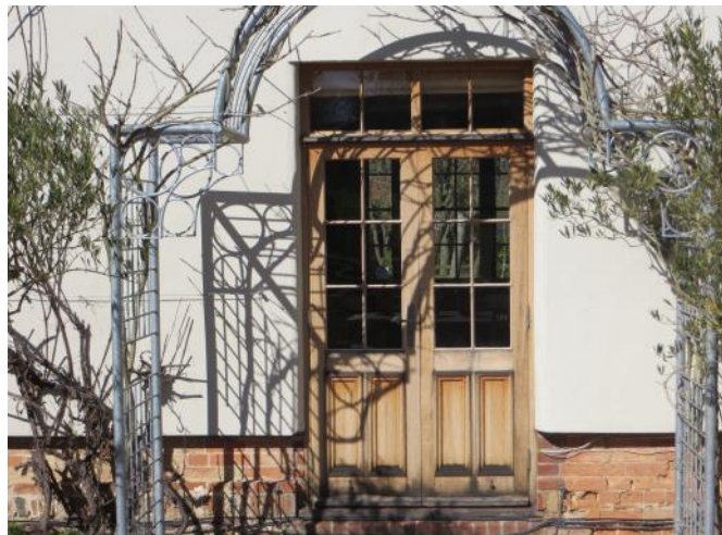
Figure 4.78: Showing the French doors on the southern elevation of the main range.
