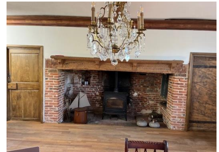
Figure 4.104: Showing the dining room's historic fireplace bressummer on the western wall of the room.
