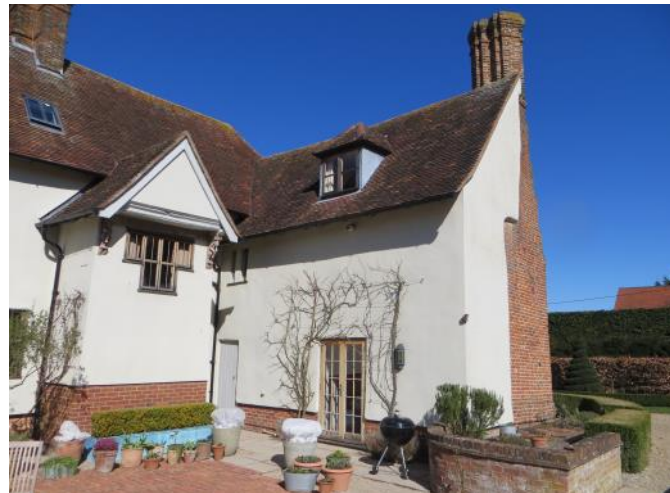
Figure 4.67: Showing the western elevation of the kitchen cross wing.
