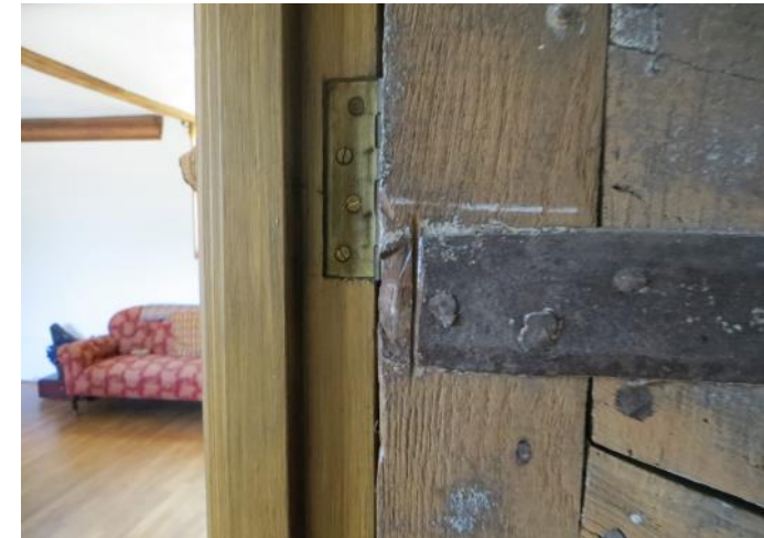
Figure 4.89: Showing the historic remnants of strap hinges on the dining room side of the 3-plank door.
