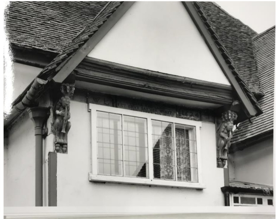
Figure 4.8: 1992-94 photograph showing the first floor window in the rear stair wing (Source: Historic England Archives).
