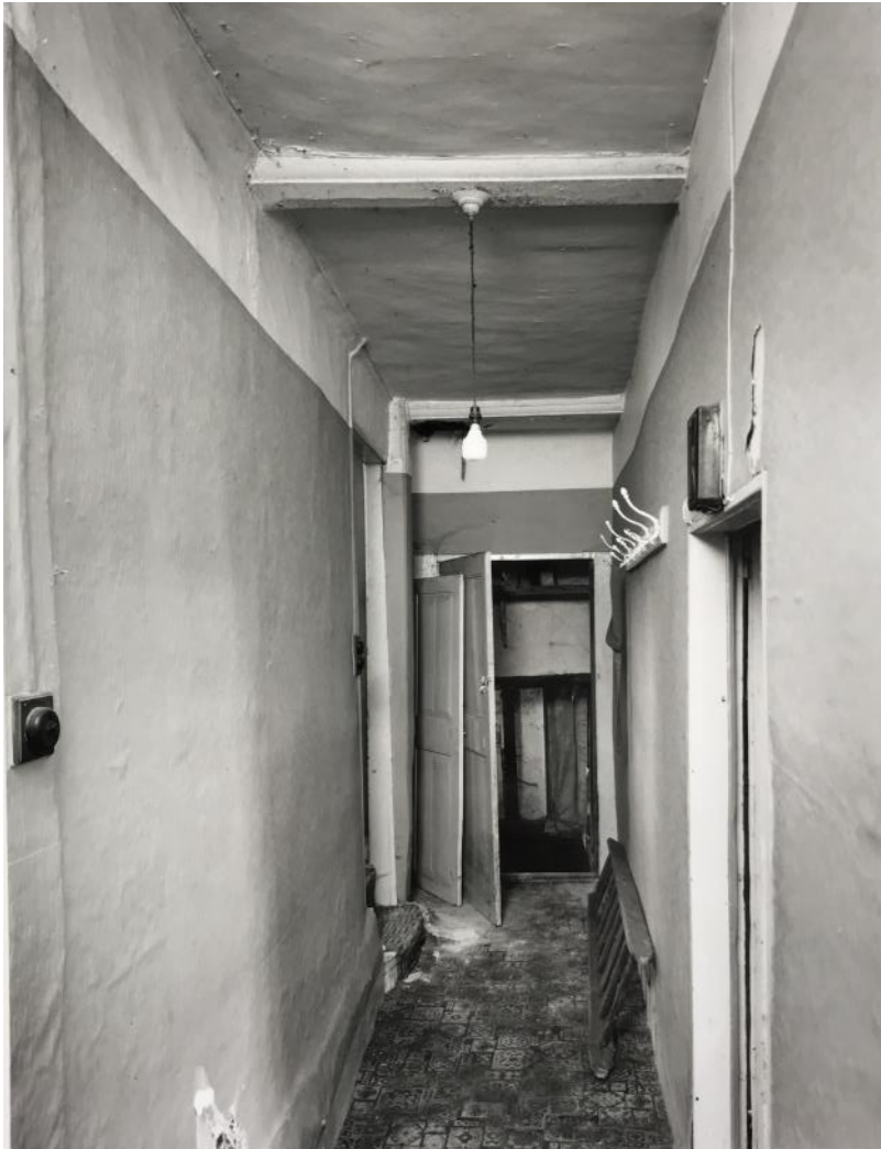
Figure 4.13: 1992-94 photograph showing the ground floor corridor that used to run along the southern side of the dining room looking west (Source: Historic England Archives, Reference: BB92/06146). Note the steps up to the stair wing on the left hand side.
