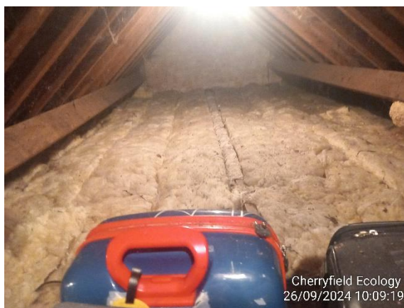
Figure 6: Example of B1's loft void
