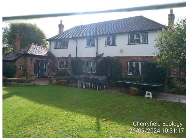
Figure 3: Example of B1's exterior
