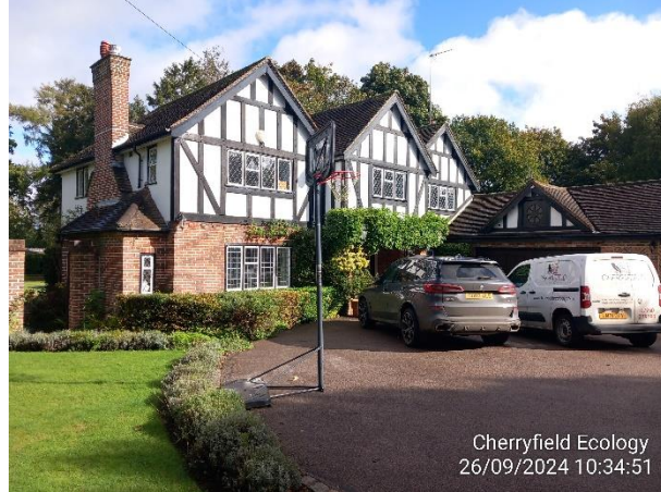
Figure 2: Example of B1's exterior
