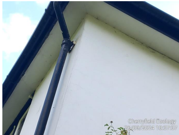
Figure 10: Example of the tight soffit box
