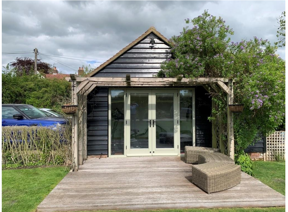
Photo of french doors inserted into side elevation of the garage building to provide natural light
