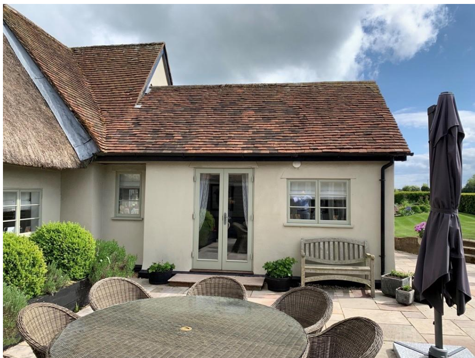
Photo of side elevation of the 1985 and 2021 extension taken from courtyard. Use of materials matching the 1985 extension provides a seamless minor change
