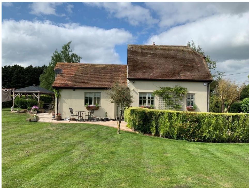
Photo of side elevation of the 1985 and 2021 extension taken from garden. Note the matching materials providing a seamless minor change
