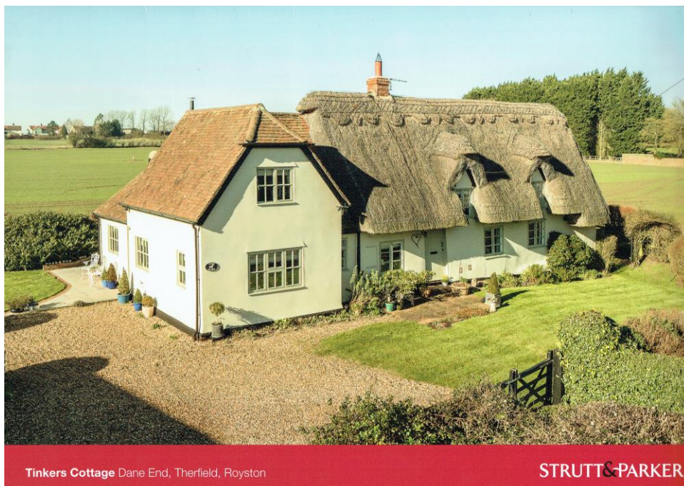
Front page of Sale brochure dated 2016. Note the same appearance of windows and front door in 2016 to that installed in 2018 and 2019
