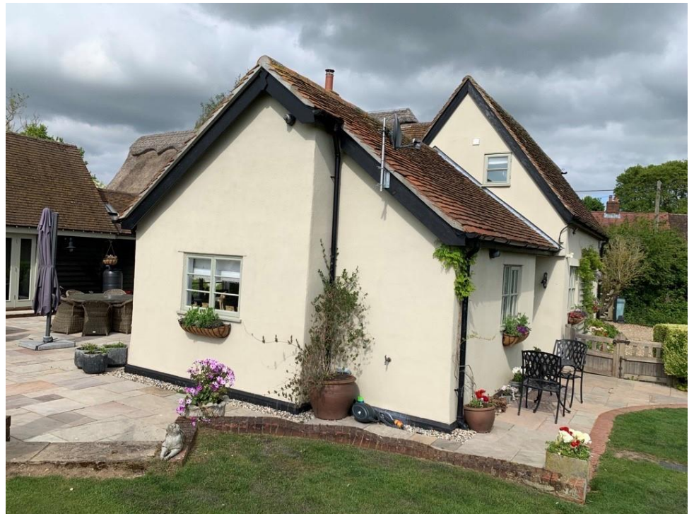
Photo of the rear of the 2021 extension. Note the use of materials to match to provide a seamless alteration.
