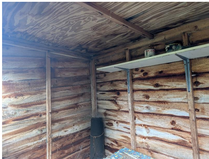
Figure 15: Interior of timber shed
