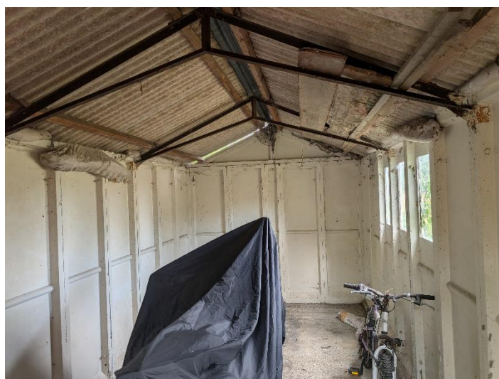
Figure 13: Interior of garage
