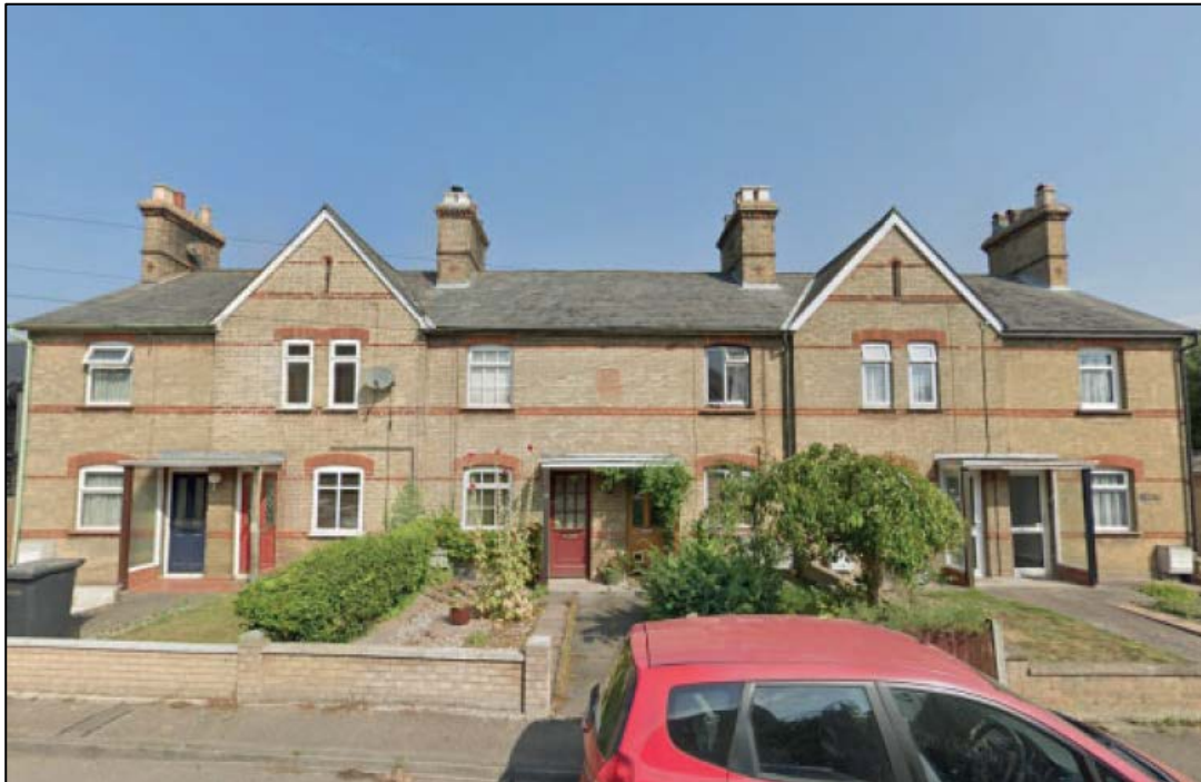
Figure 2 - Victorian Terrace 2-12 Shillington Road, Pirton
