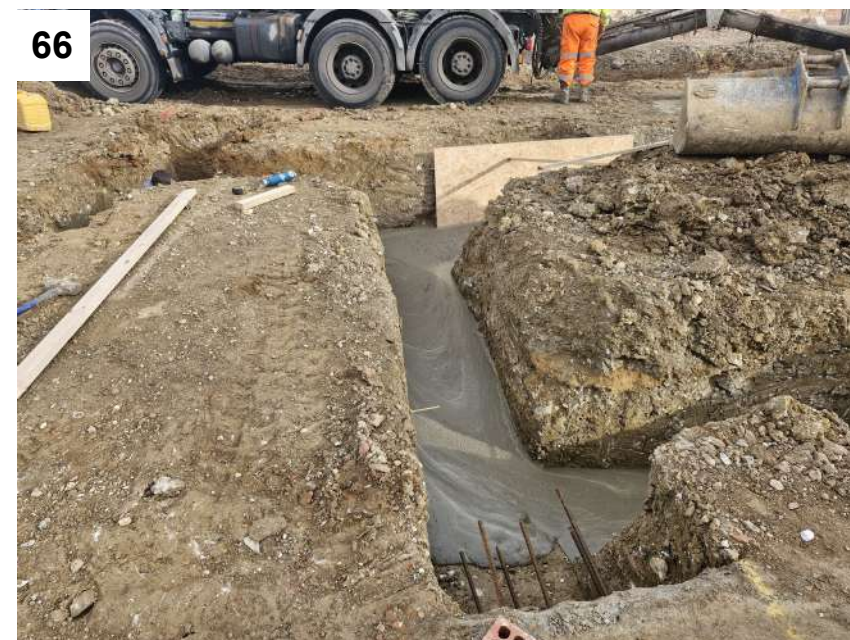
Photos 65 & 66 — View of concrete being poured into the footings with an MDF wood board covering the hydrocarbon stained area to help this material be excavated further later.
