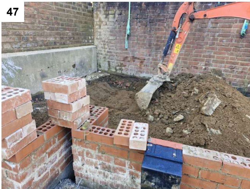
Photos 47 to 50 — View of the excavation of the contaminated soils hotspot in the south west corner of the site
