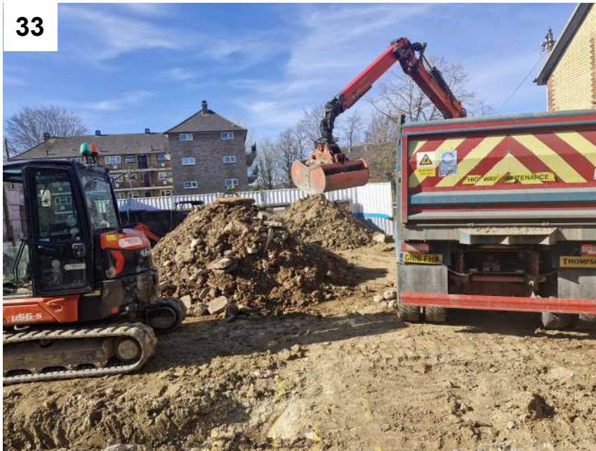
Photos 33 to 35 — View of hazardous concrete disposal with associated disposal ticket and consignment note.
