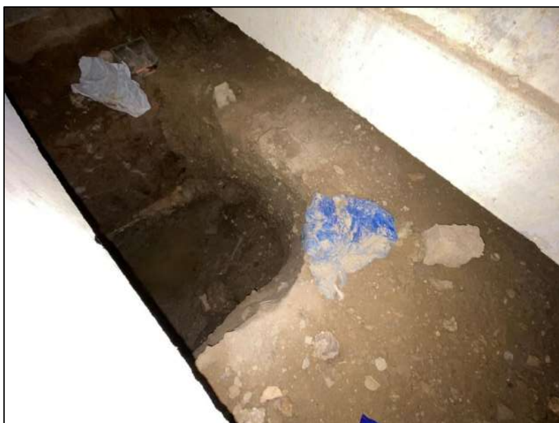
Figure 8-A: Subfloor void
