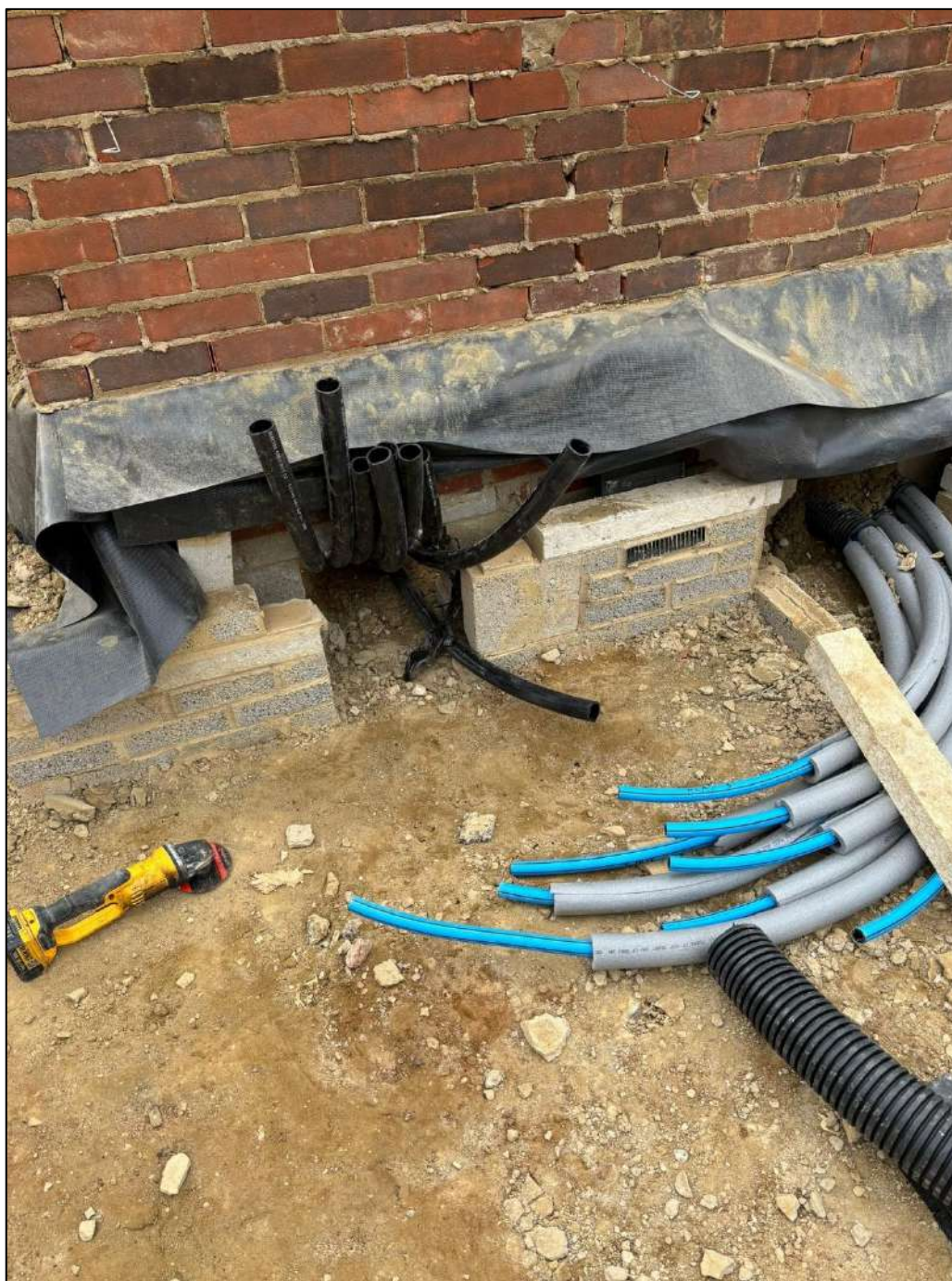
Figure 9-B: Example of protective barrier pipe installation
