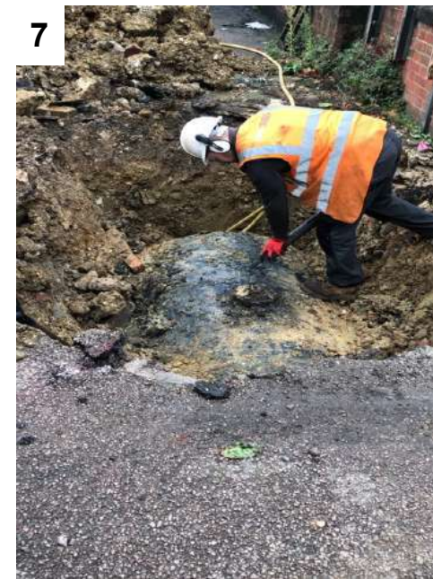
Photos 5, 6 & 7 — Excavation of the below ground fuel storage tank identified adjacent to the western site boundary
