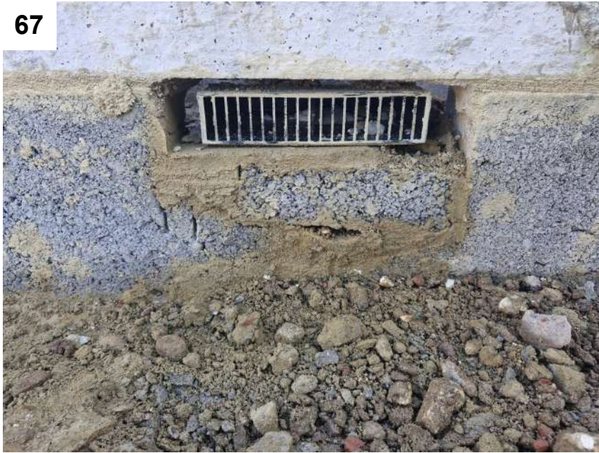
Photos 67 & 68 — View of some passive subfloor ventilation evidence observed during construction.
