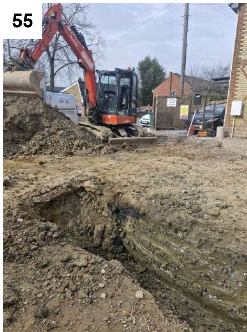
Photos 55 to 58 — View of the hydrocarbon stained material identified within the foundation trench between flats 1 and 2 with samples from that area SS01.
