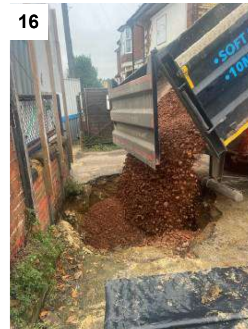
Photos 11 to 16 — View the tank being removed, the resulting excavation, Validation samples from beneath the tank and of the backfill material; and the excavation being backfilled.
