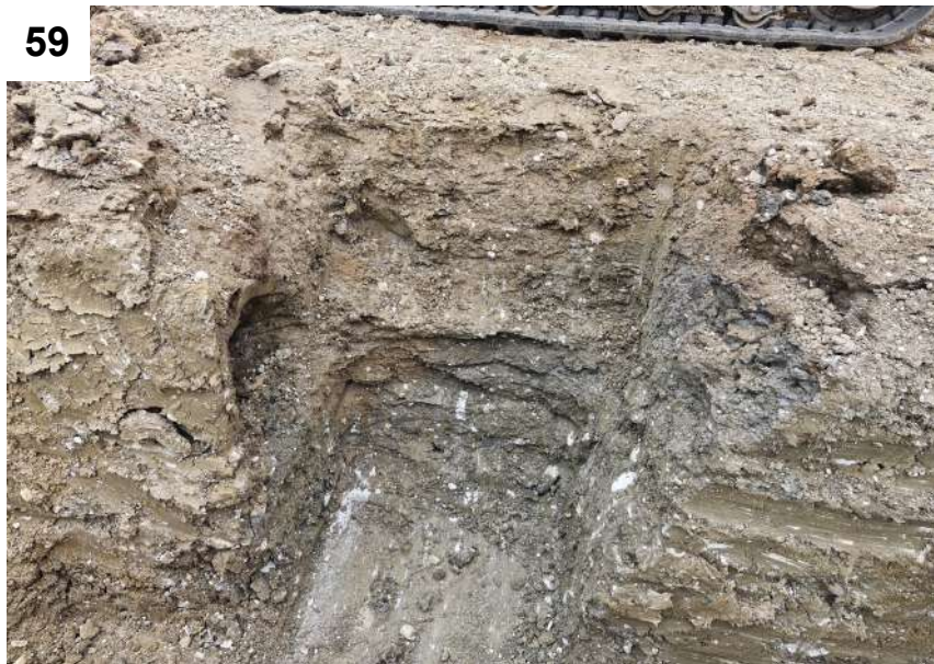
Photos 59 to 62 — View of the remedial excavation of the hydrocarbon impacted material identified within the foundation trench between flats 1 and 2 with validation samples SS01A to SS01D conducted.
