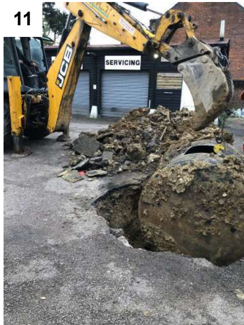
Photos 11 to 16 — View the tank being removed, the resulting excavation, Validation samples from beneath the tank and of the backfill material; and the excavation being backfilled.
