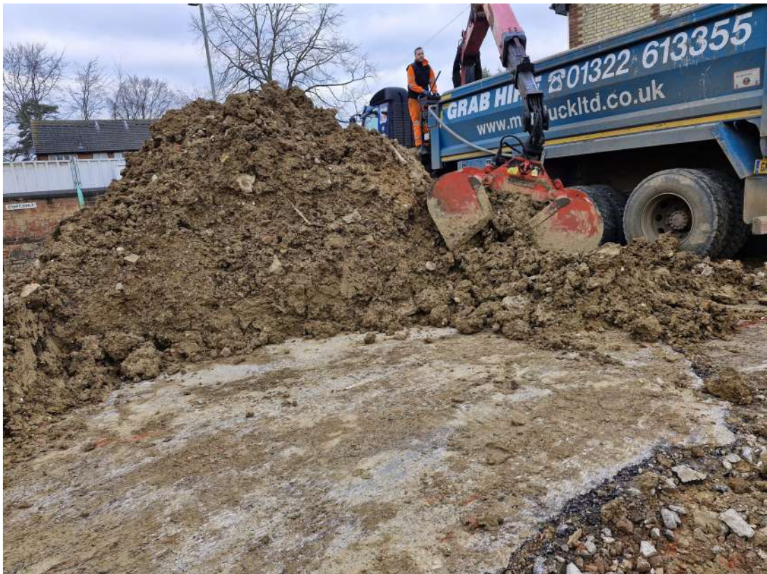
Photo 2: Showing the removal of Non-Hazardous waste.
