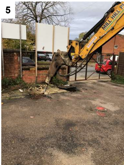
Photos 5, 6 & 7 — Excavation of the below ground fuel storage tank identified adjacent to the western site boundary
