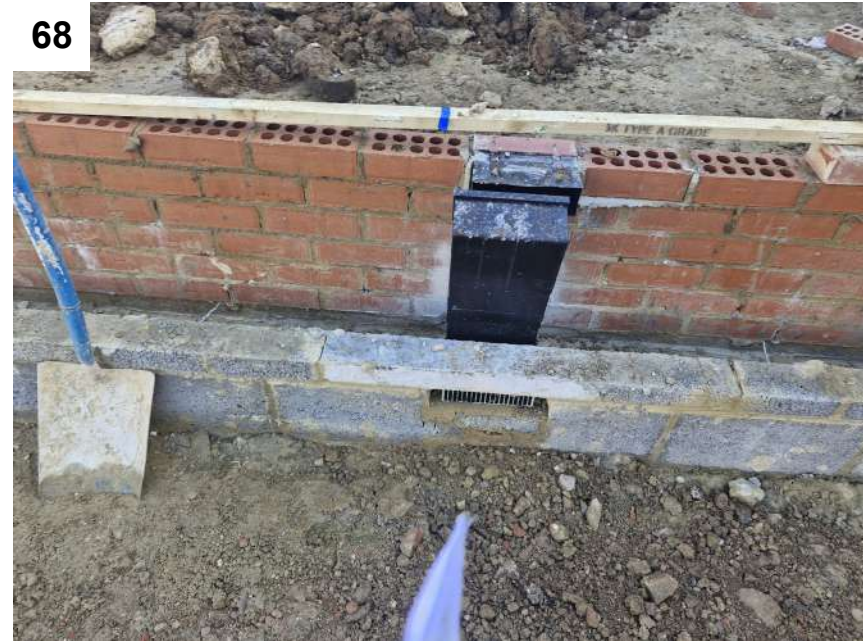
Photos 67 & 68 — View of some passive subfloor ventilation evidence observed during construction.
