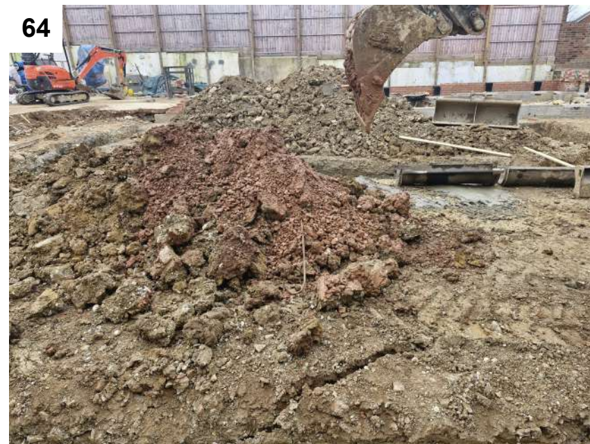
Photos 63 & 64 — View of the pink MOT excavated where the former diesel tank used to be during the foundation excavation.
