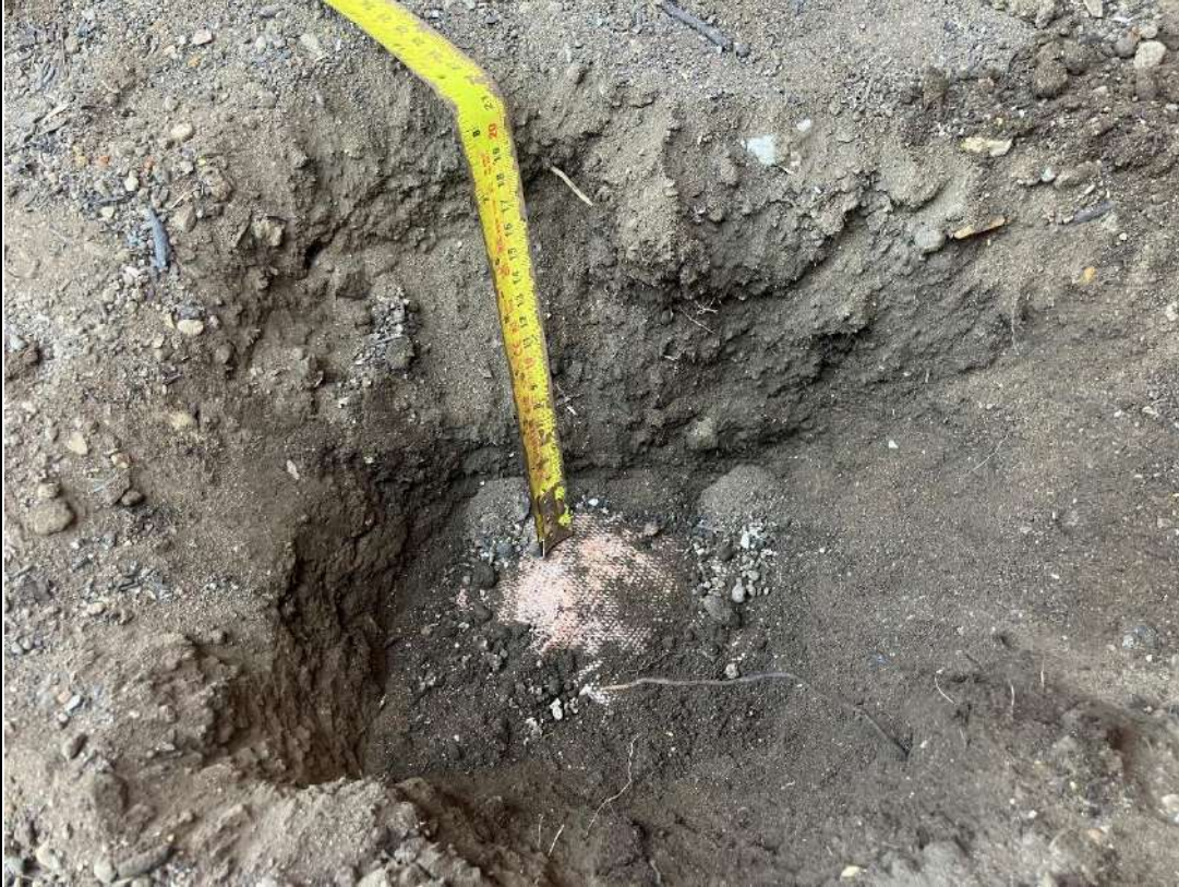
P7 – Example of soils and geotextile membrane at the base
