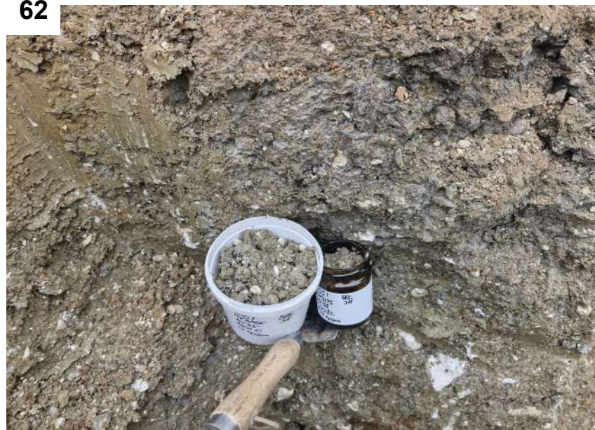
Photos 59 to 62 — View of the remedial excavation of the hydrocarbon impacted material identified within the foundation trench between flats 1 and 2 with validation samples SS01A to SS01D conducted.
