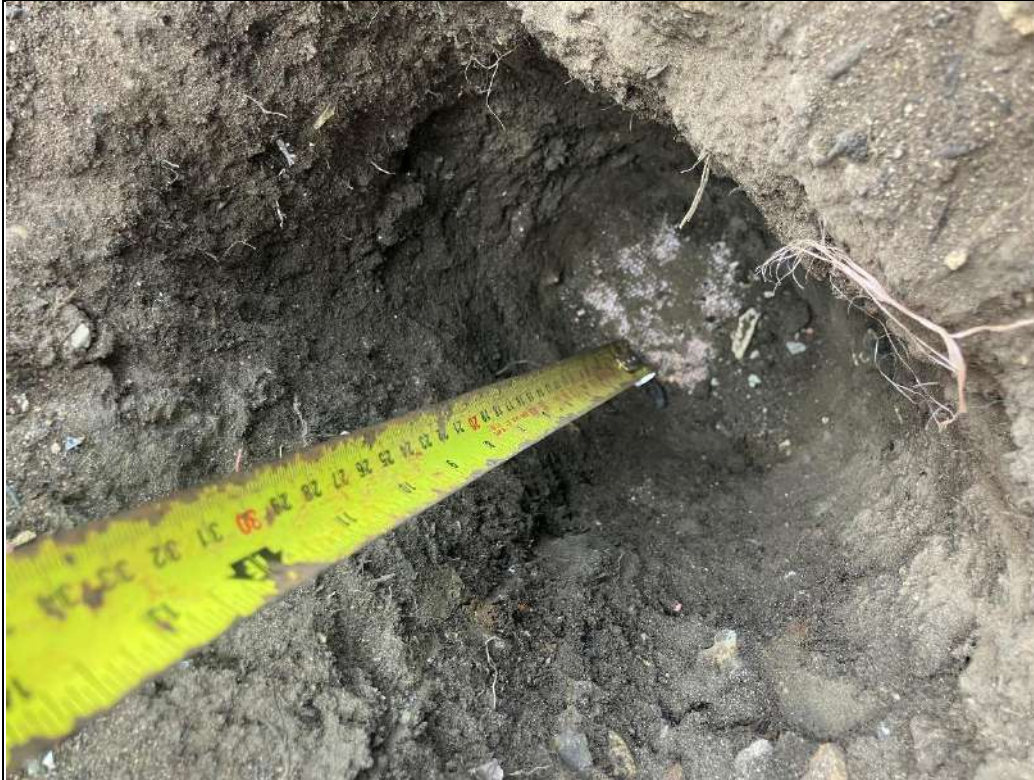
P3 – geotextile membrane at 0.30m bgl
