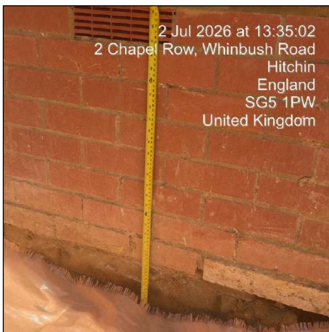
Figure 7-C: Example of geotextile membrane placement
