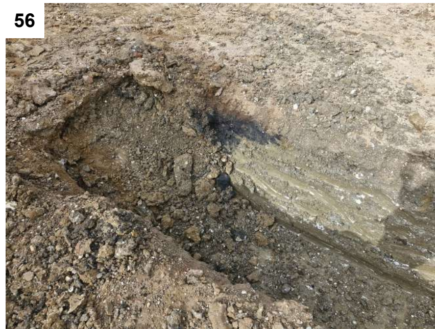
Photos 55 to 58 — View of the hydrocarbon stained material identified within the foundation trench between flats 1 and 2 with samples from that area SS01.
