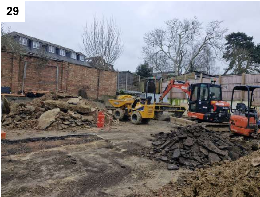
Photos 29 & 30 — Example of stockpile segregation during SEC's watching brief.
