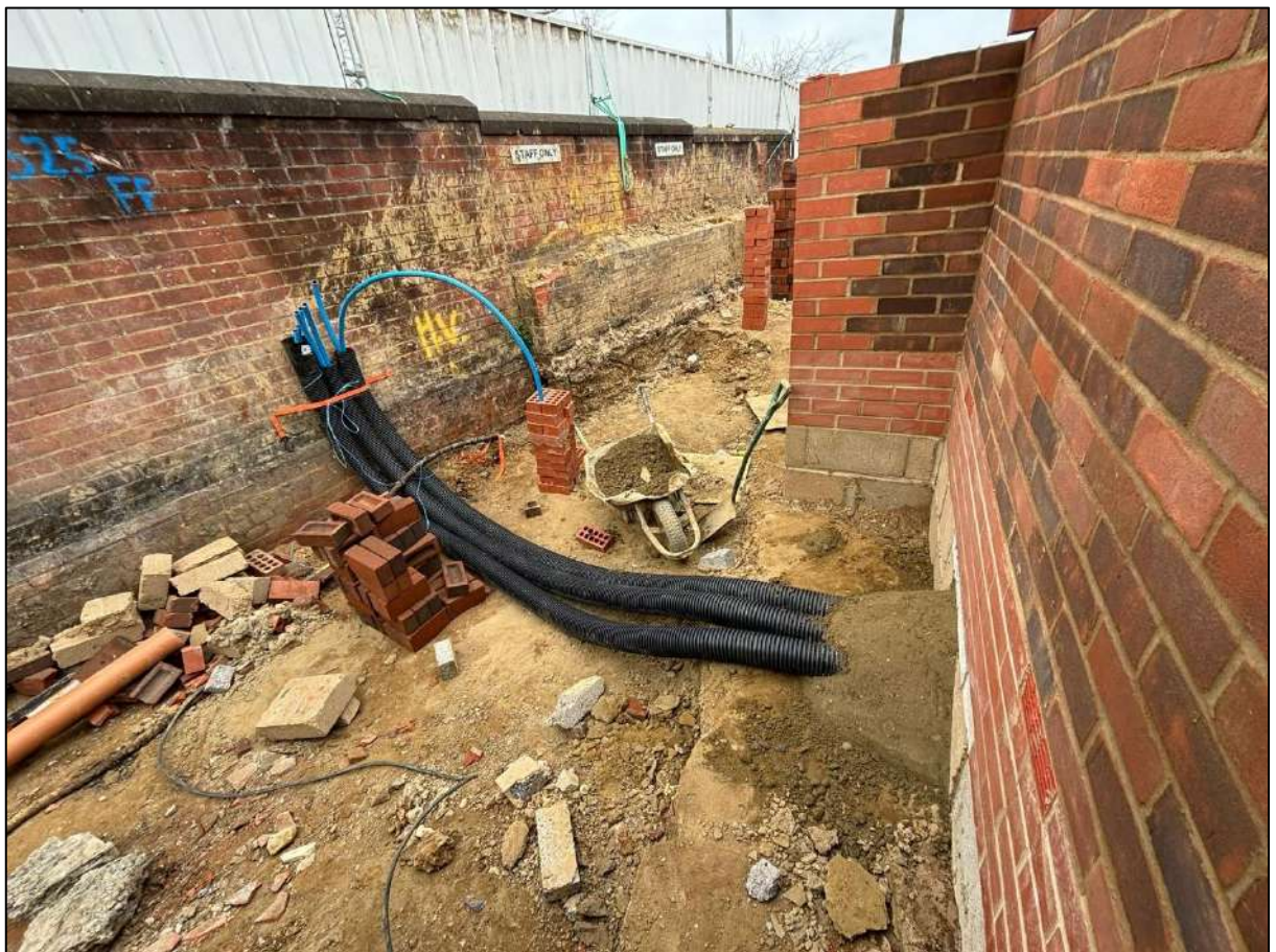
Figure 9-A: Spatial photograph of barrier pipe installation
