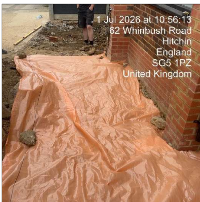
Figure 7-B: Example of geotextile membrane placement
