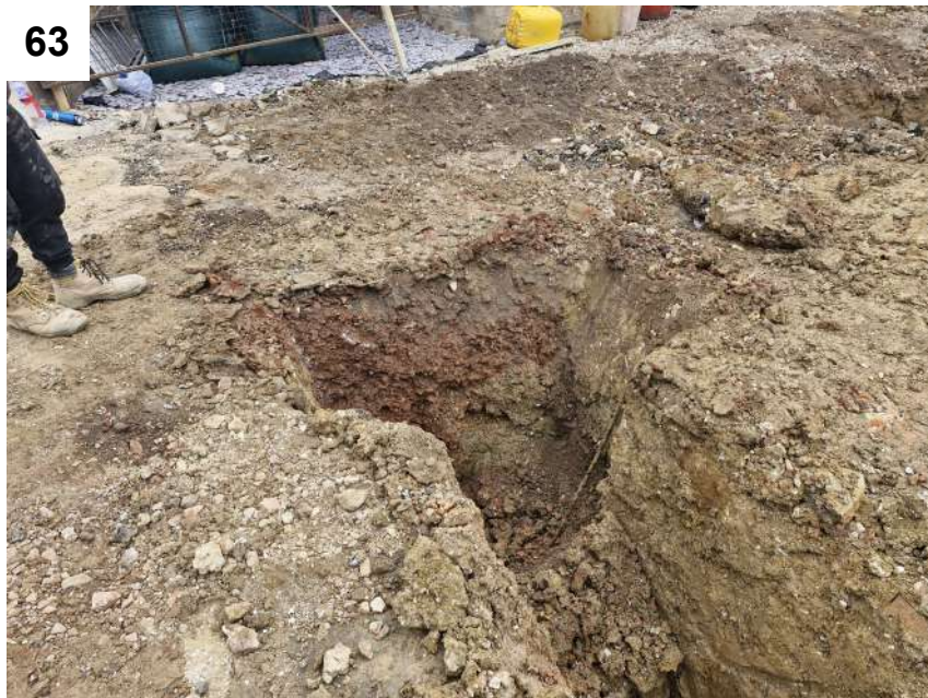
Photos 63 & 64 — View of the pink MOT excavated where the former diesel tank used to be during the foundation excavation.
