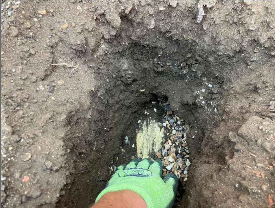
P1 – geotextile membrane at 0.30m bgl
