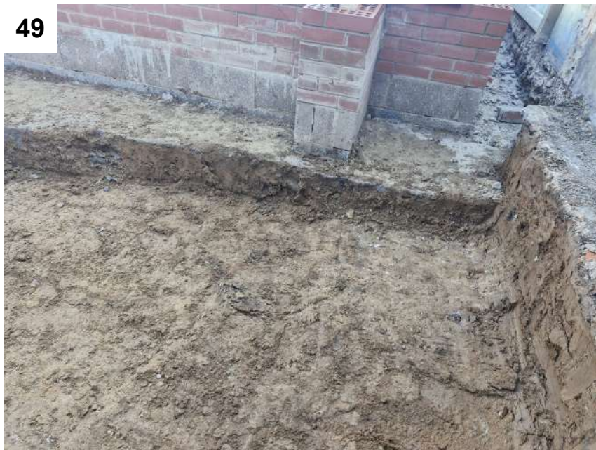
Photos 47 to 50 — View of the excavation of the contaminated soils hotspot in the south west corner of the site
