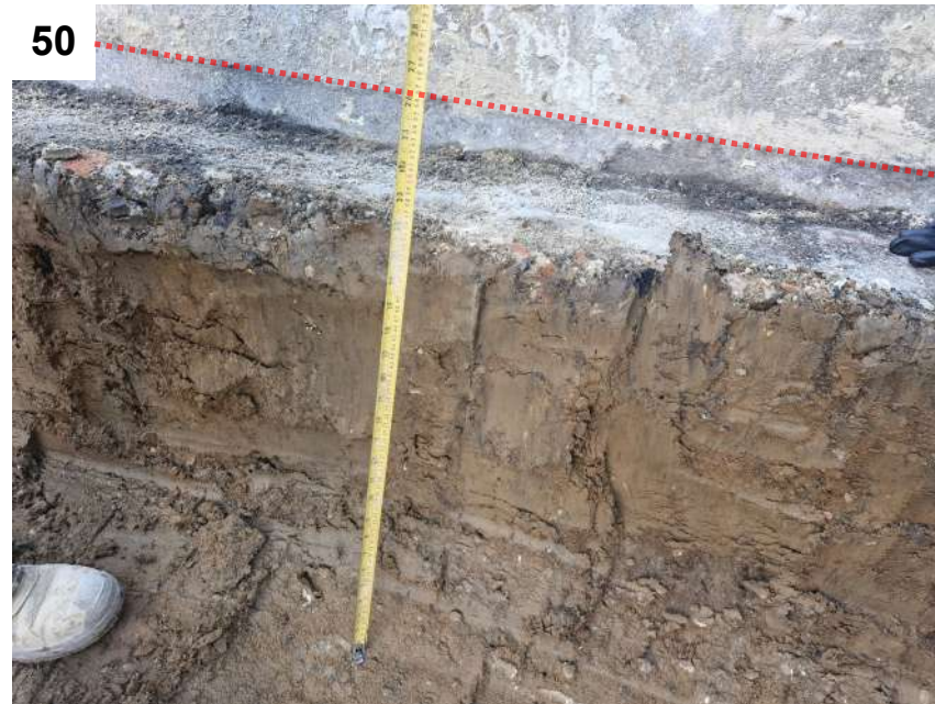
Photos 47 to 50 — View of the excavation of the contaminated soils hotspot in the south west corner of the site
