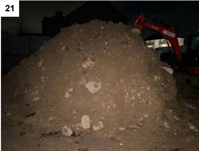
Photos 21 & 22 — View of arising stockpiles entrained with tarmac observed on 30/01/2025 prior to SEC's commencement of the Watching Brief.
