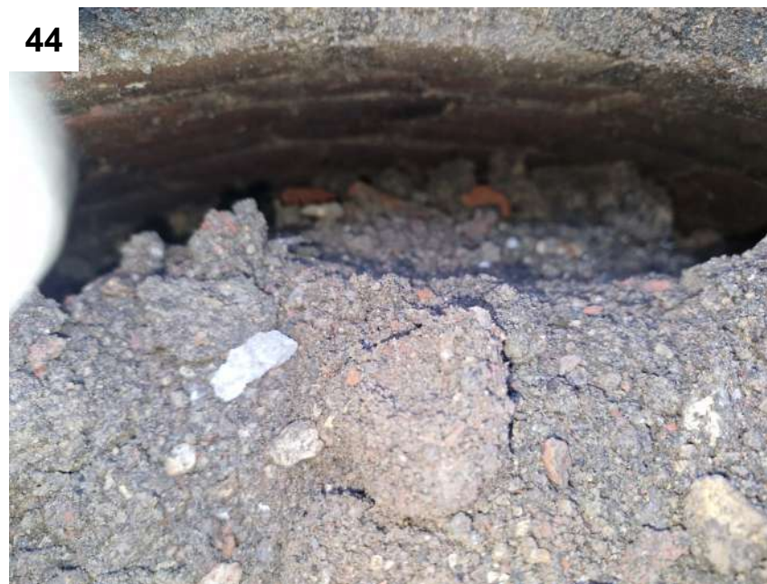
Photos 43 to 46 — View of the infilled soakaway feature identified to the western side of the site, the infill material and associated sampling - Val01.
