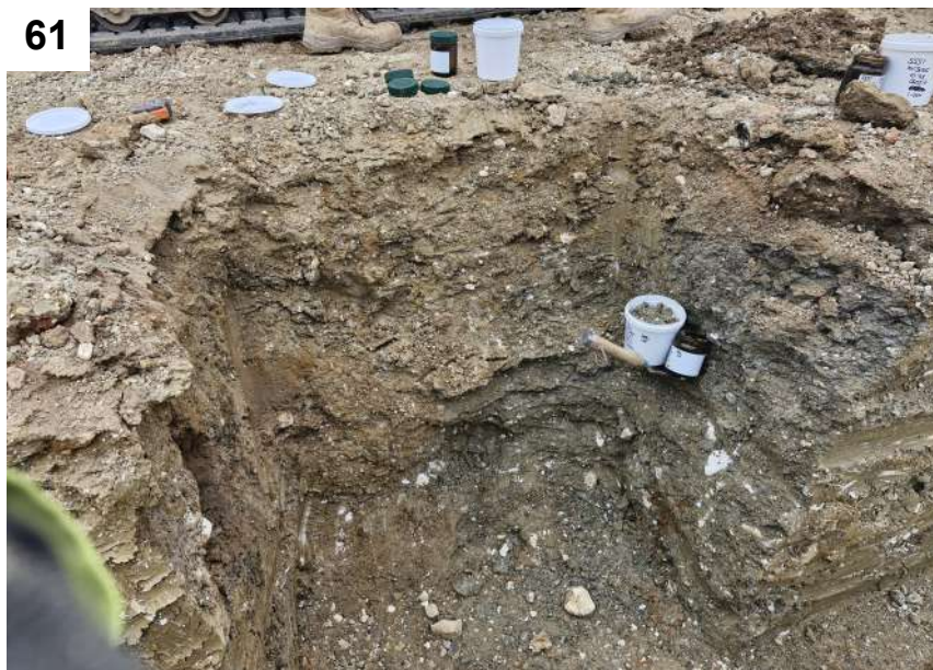
Photos 59 to 62 — View of the remedial excavation of the hydrocarbon impacted material identified within the foundation trench between flats 1 and 2 with validation samples SS01A to SS01D conducted.
