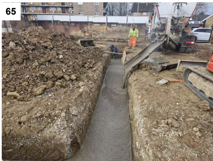
Photos 65 & 66 — View of concrete being poured into the footings with an MDF wood board covering the hydrocarbon stained area to help this material be excavated further later.
