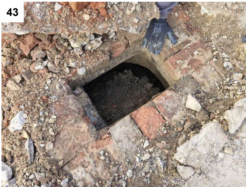
Photos 43 to 46 — View of the infilled soakaway feature identified to the western side of the site, the infill material and associated sampling - Val01.
