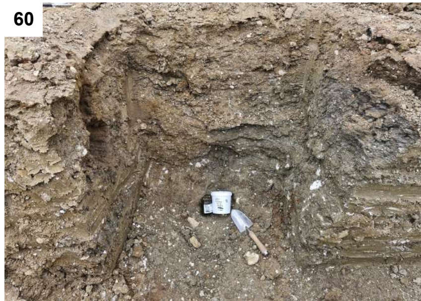
Photos 59 to 62 — View of the remedial excavation of the hydrocarbon impacted material identified within the foundation trench between flats 1 and 2 with validation samples SS01A to SS01D conducted.
