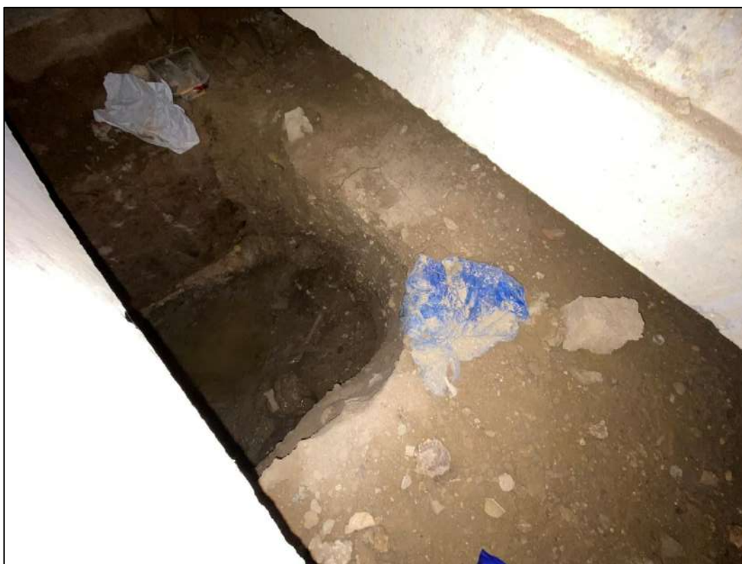
Figure 3-A: Excavation under building footprint
