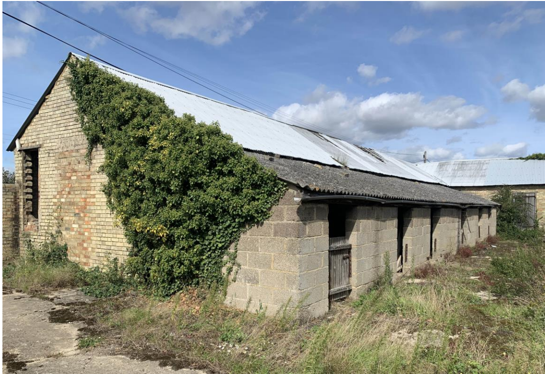
Figure 9. South and east elevations of west wing
