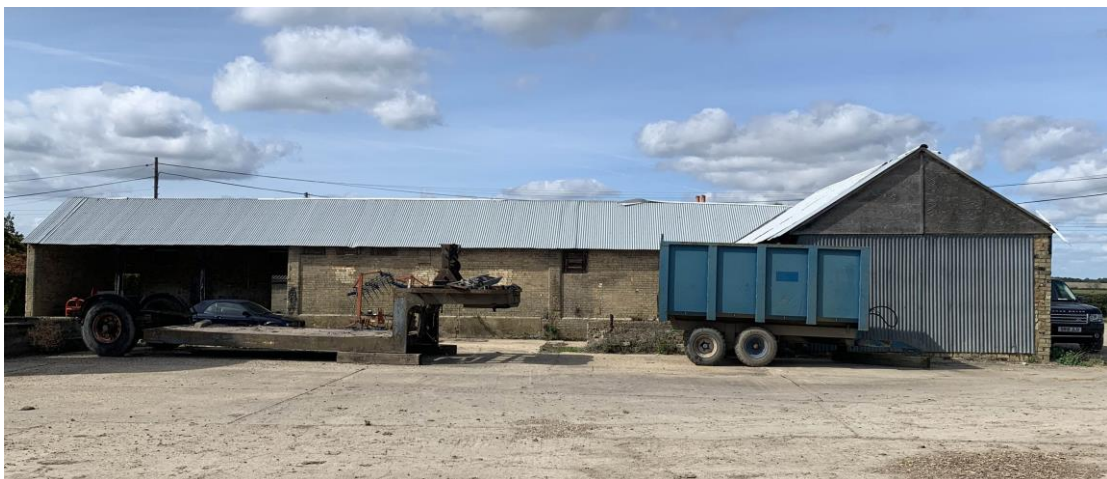
Figure 8. East elevation of east wing
