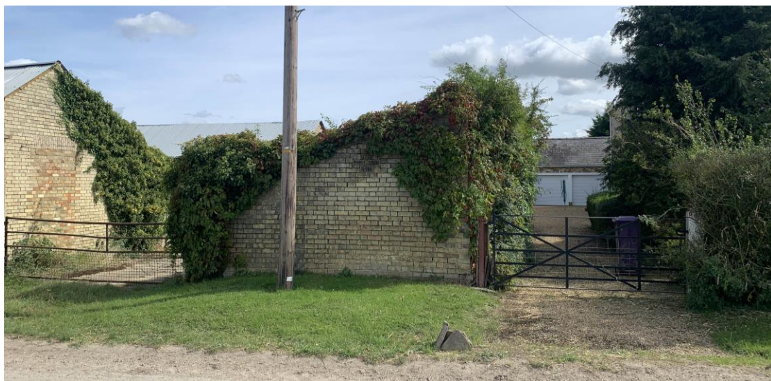
Figure 12. West elevation (Northfield Road)
