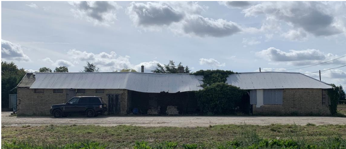
Figure 7. North elevation of north wing
