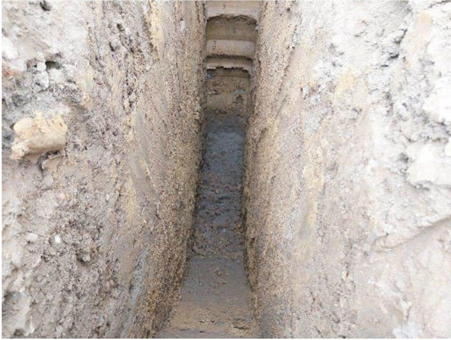
Photograph 1 - Looking down within TP01.
