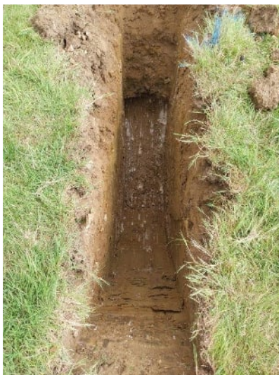
Photograph 5 - Looking down within TP03.
