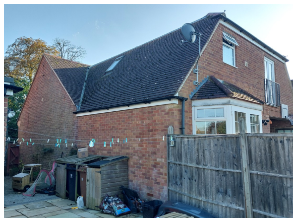
Fig. 7. Existing extension at 29 Turnpike Lane.
