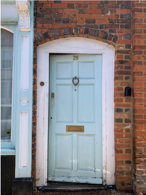
Existing s/w front door
