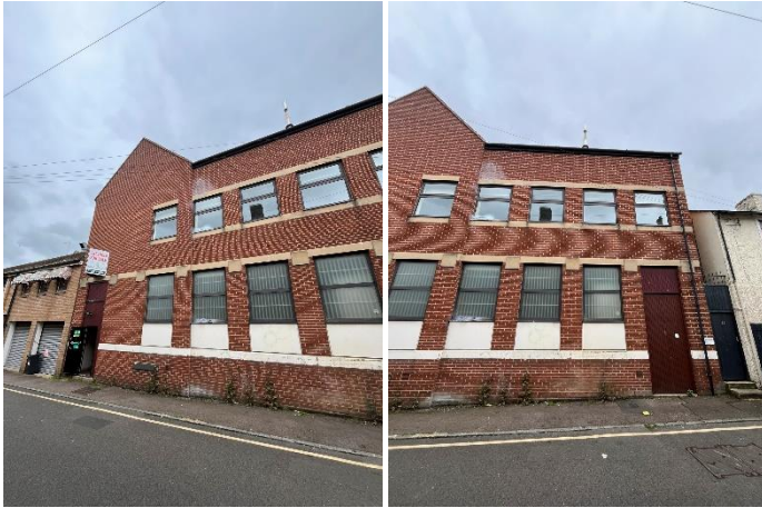
Rear elevation from Kings Street
