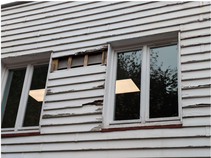
Image showing the modern materials to be replaced.
