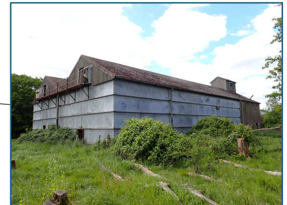
VIEW SOUTHWEST OF GRAINSTORE
