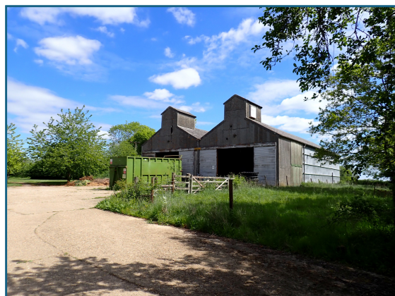
VIEW NORTHEAST OF GRAINSTORE
