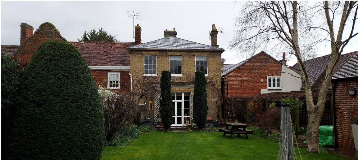
Rear elevation – openings 5, 11-13
