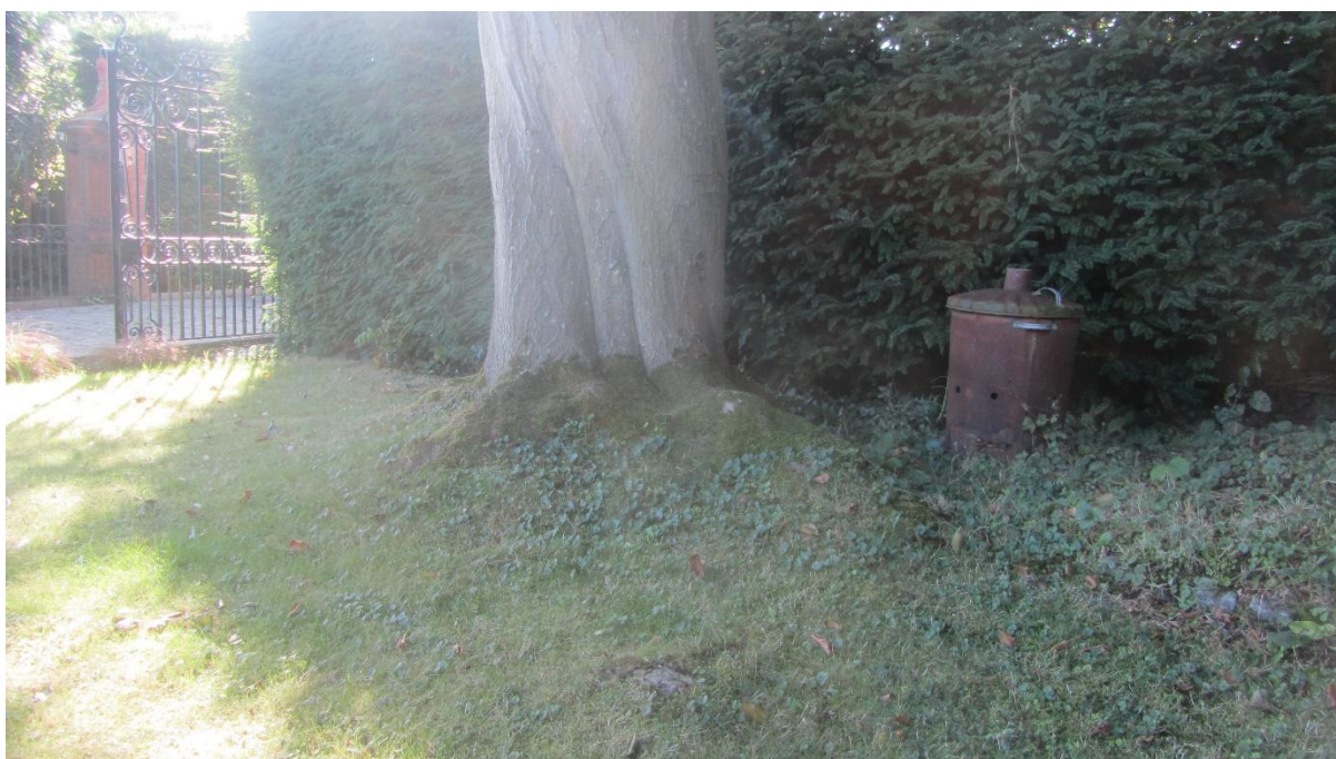
PHOTOGRAPH NO. 8 – Northwest side of the base of T2
