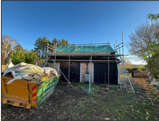
Fig 4 – Front elevation of the existing out-building.
