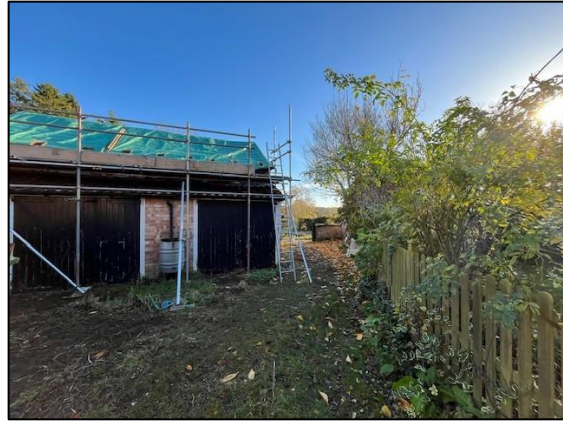
Fig 5 – Front elevation and adjacent neighbour's garden.
