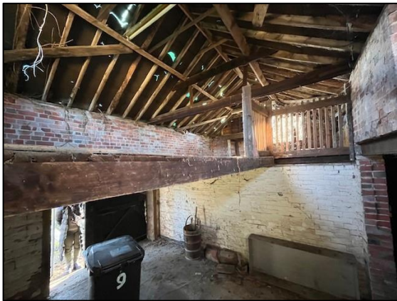
Fig 12 – General internal view looking north.
