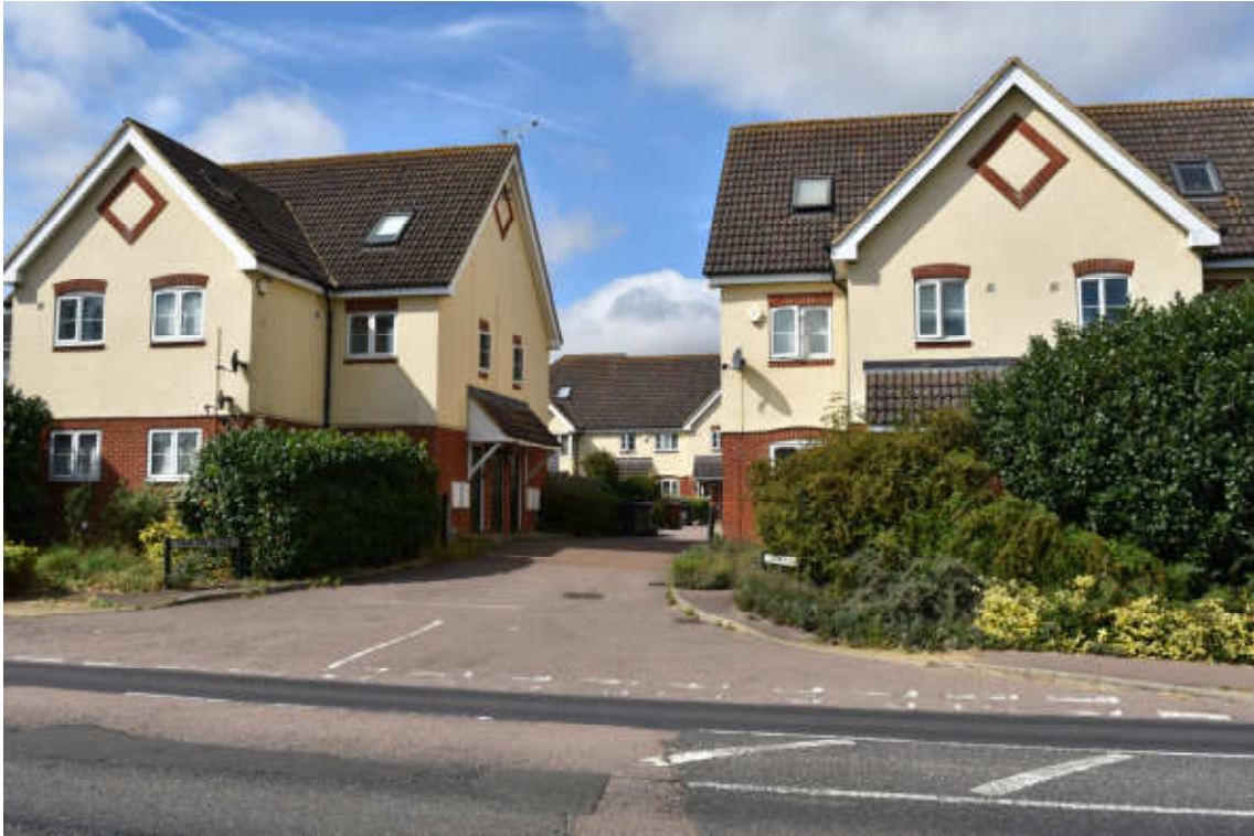
Photograph 4 Typical late 20 th century infill at Westmill where the original layout was lower density.
