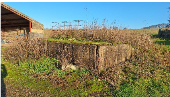
PLATE 10: CONCRETE STRUCTURE TO EAST
