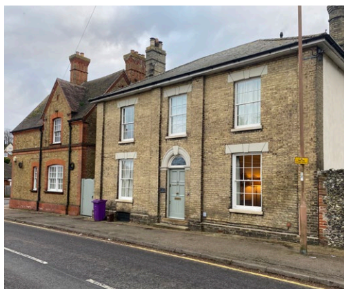
GEORGIAN BUILDING ON MARKET HILL
