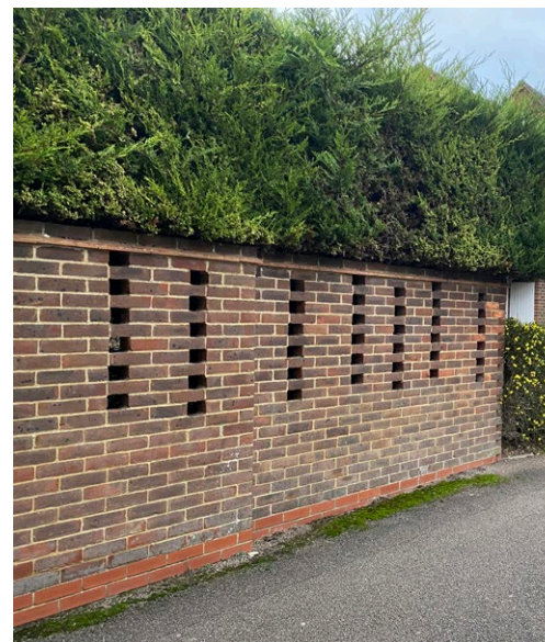
HIGH BRICK WALL WITH DETAILING
