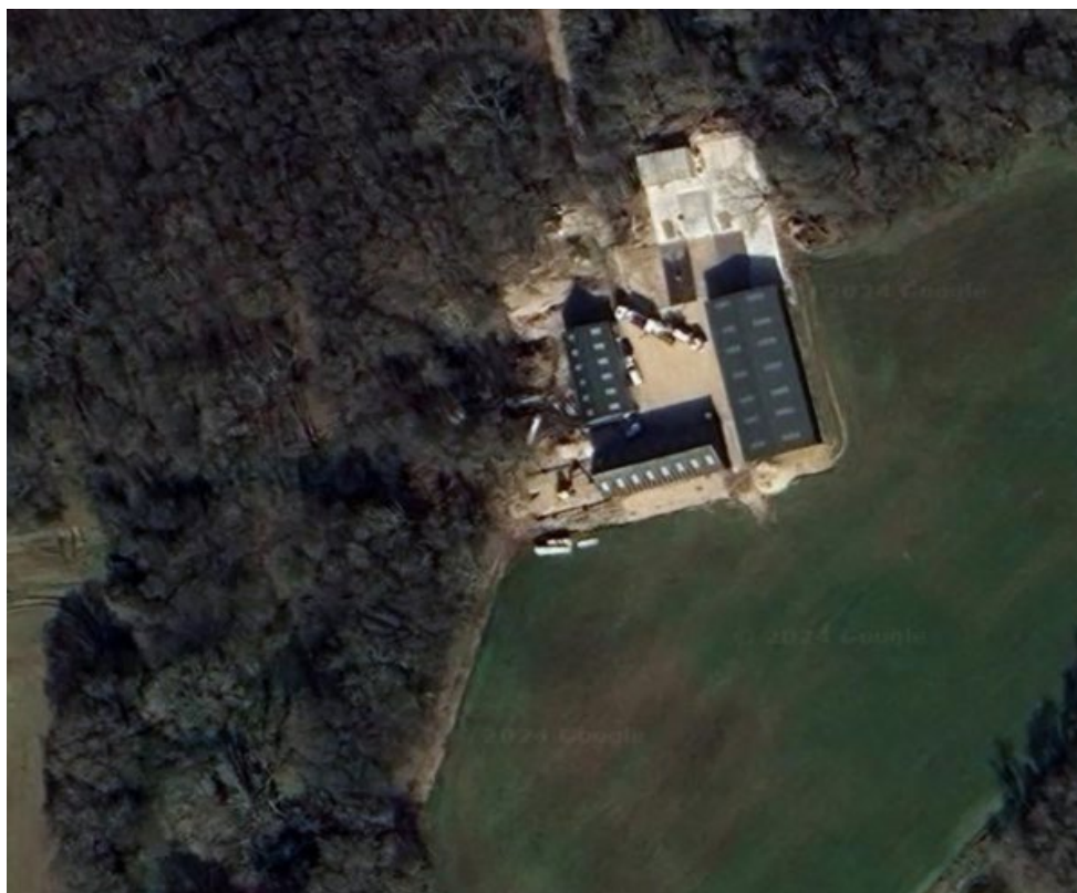
Figure 17: Aerial image of the application site showing Barn design.
