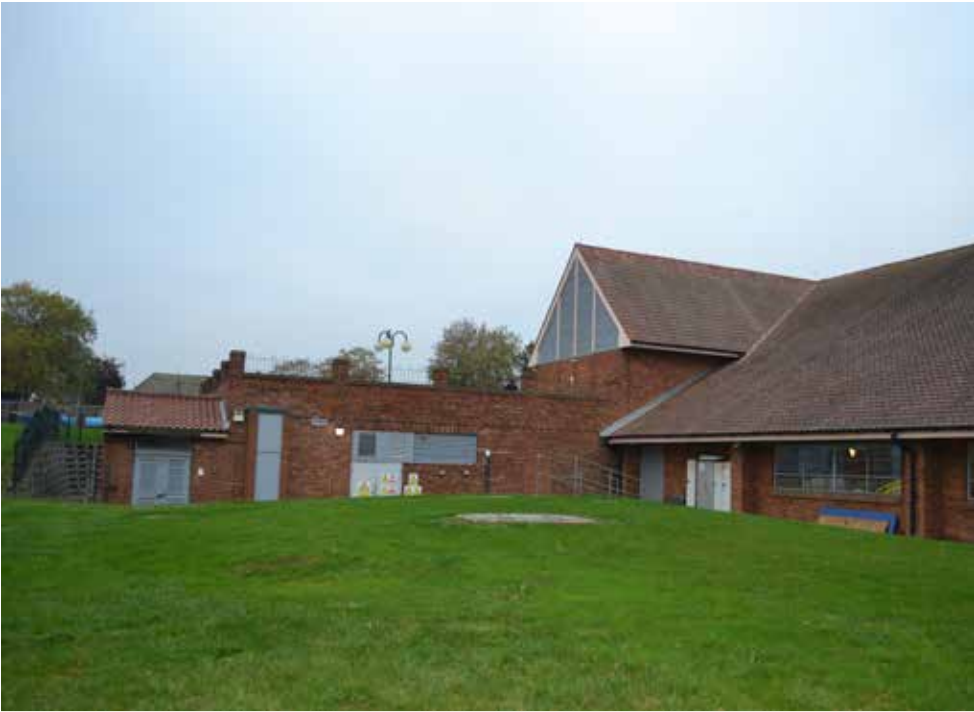
Figure 11 - View of the building from the south, within the site boundaries.
