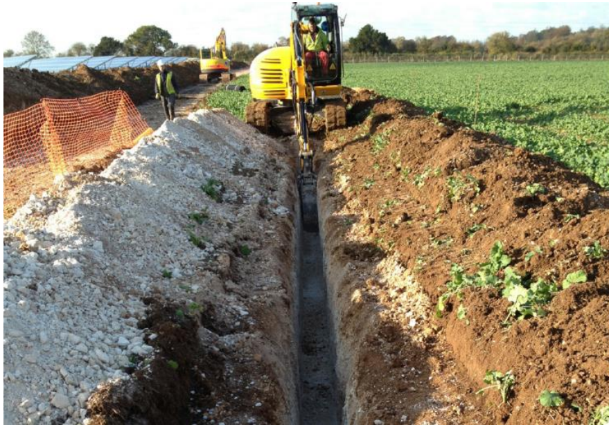
Figure 1: Example of cable trenching with separations of soils; topsoil stripped and placed on the right, subsoil on the left (Copyright CRE, 2014).
