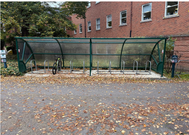
FIGURE 2.5.1 - EXISTING CYCLE SHELTER
