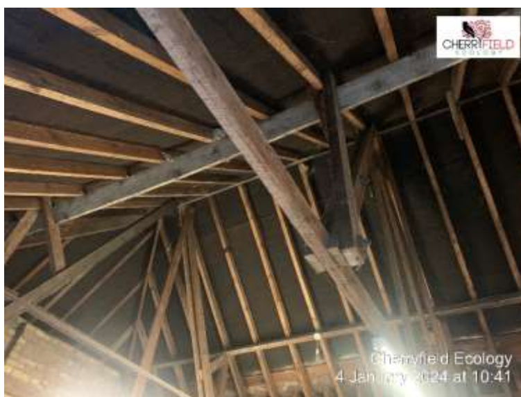
Figure 10: Another example of the interior of the garage attached to B1.
