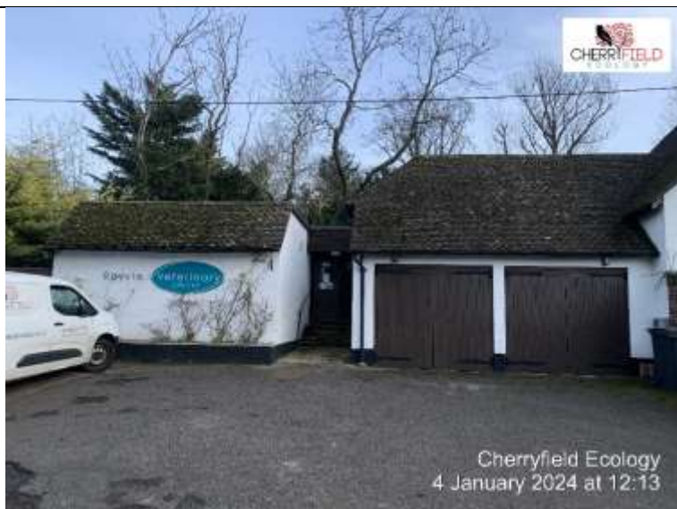
Figure 5: Front view of garage and extension to B1.
