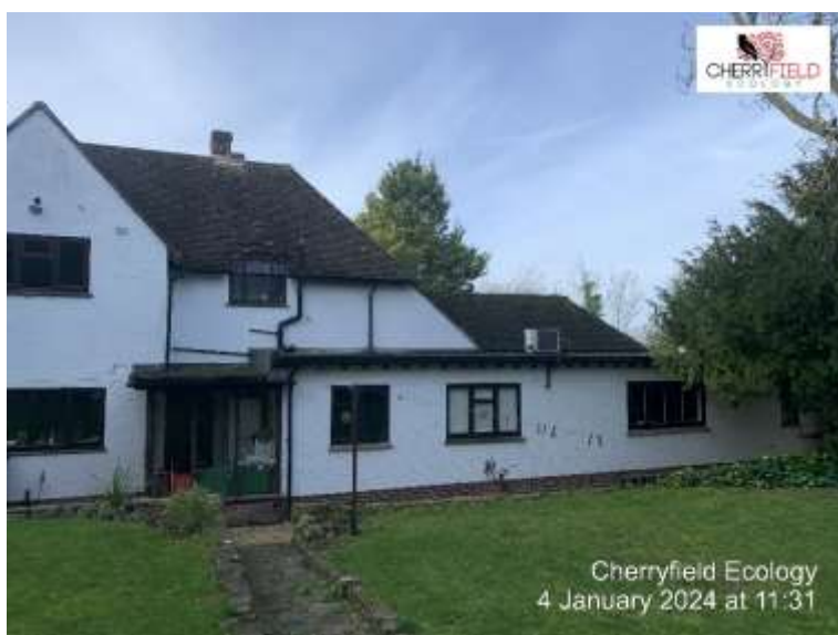
Figure 6: Rear view of garage and extension to B1.
