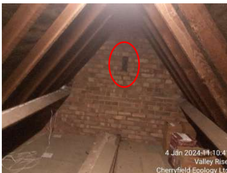
Figure 31: Air brick within the loft in the main section of B1.
