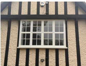
Existing External Window Elevation Image
