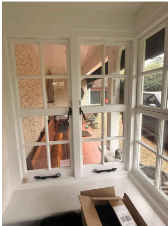
Existing Window Internally Image
