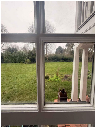
Existing Window Profile Image
