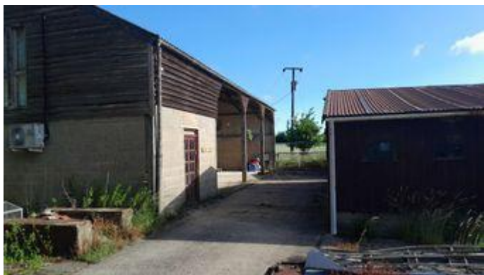
Large rectangular barn in the east of site with suspected asbestos roof and smaller rectangular barns just east of this.
