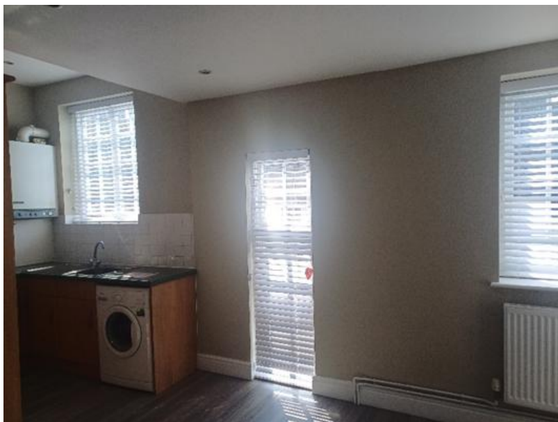
Existing internal elevation of Flat 3
