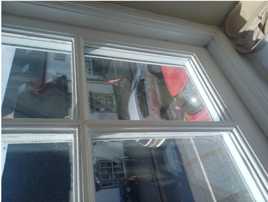
Existing internal windows 5 & 7
