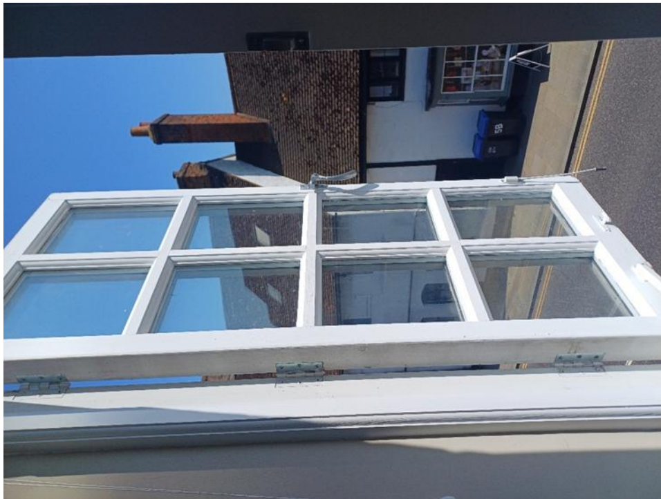
Existing Casement – openings 1-4
