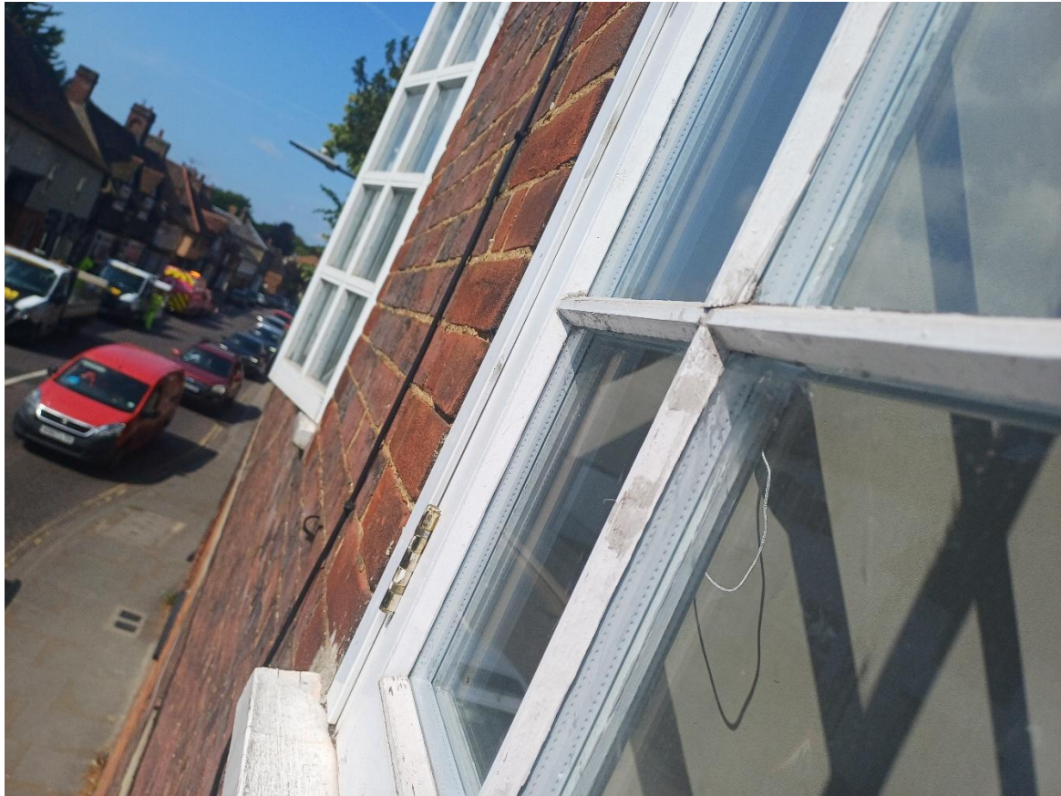
Existing external windows 5 & 7
