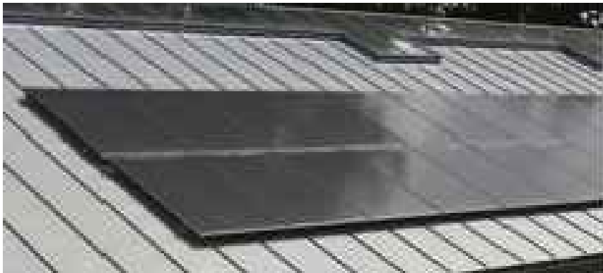
METAL STANDING SEAM ROOF – COLOUR ANTHRACITE (WITH SOLAR PANELS)
