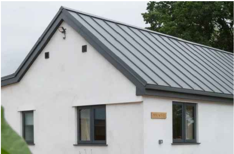
METAL STANDING SEAM ROOF – COLOUR ANTHRACITE (WITH SOLAR PANELS)
