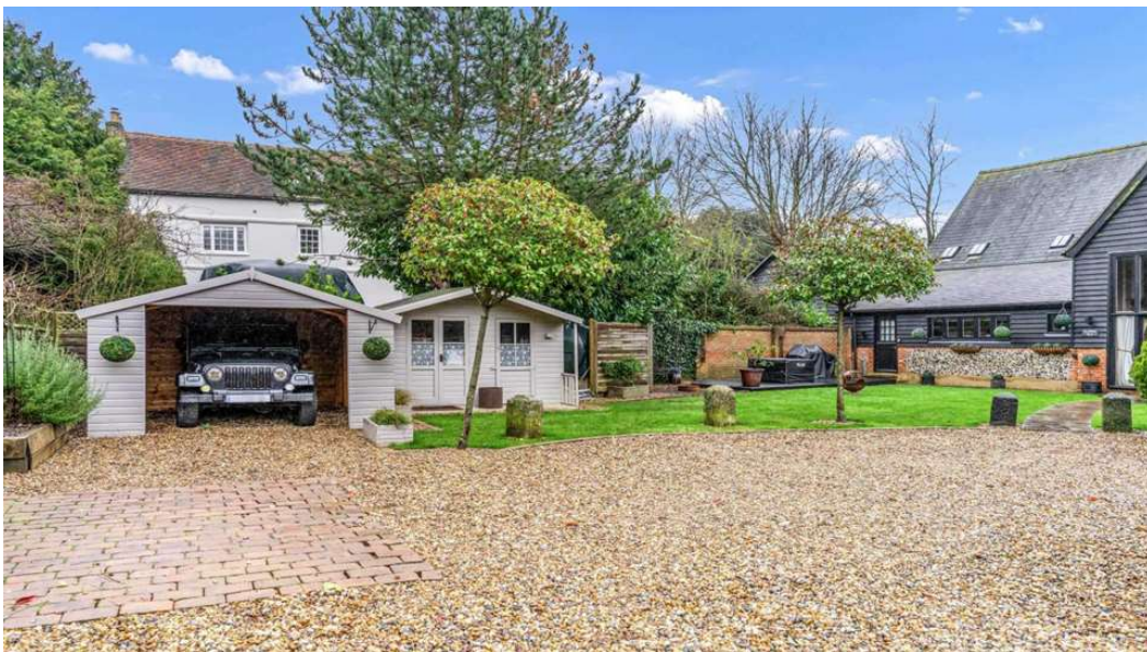
View of the north west elevation of Gannock Farmhouse from the driveway to the neighbouring Bradfield barn
