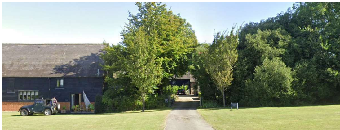
The edge of the north west elevation is briefly visible down the existing driveway.
