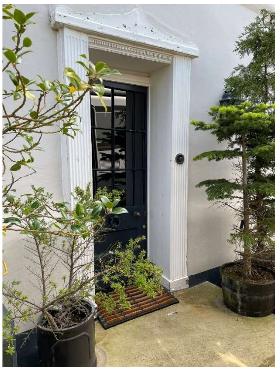
Current photograph of the entrance showing the dentil course and shallow pediment as mentioned in the listing
