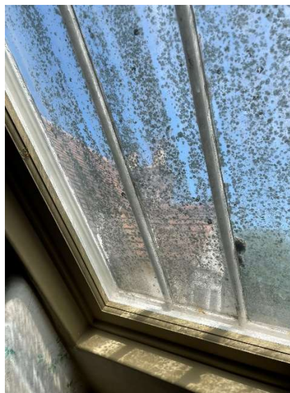
Fixed rooflight (1) just beyond the top of the stairs
