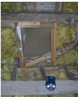
Current small access hatch
