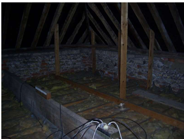
Spine beam, ceiling joists and hangers
