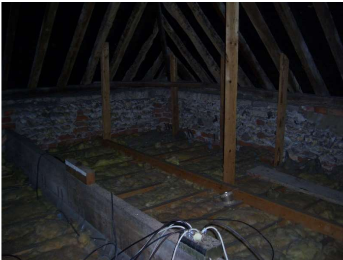
Loft space to be converted
