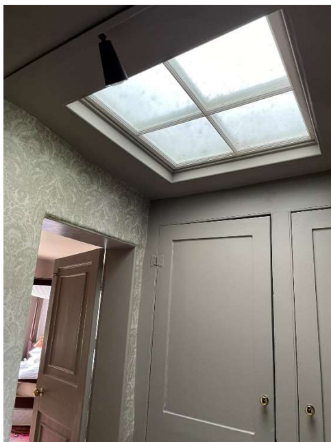
Photograph showing the glazed panel above the ceiling and the plywood shaft in the loft which links it to the rooflight
