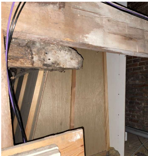
Photograph showing the glazed panel above the ceiling and the plywood shaft in the loft which links it to the rooflight
