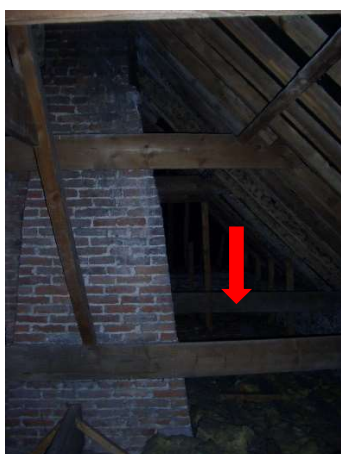
Tie beam beyond to be removed
