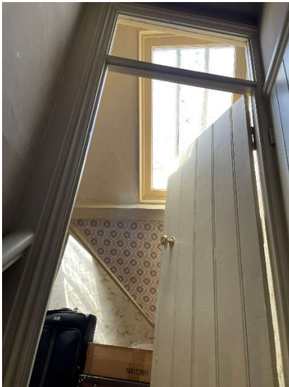
Fixed rooflight (2) at the top of the stairs
