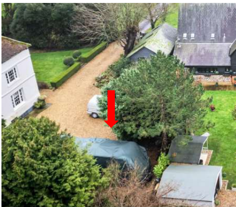
Aerial view of proposed cart lodge site
