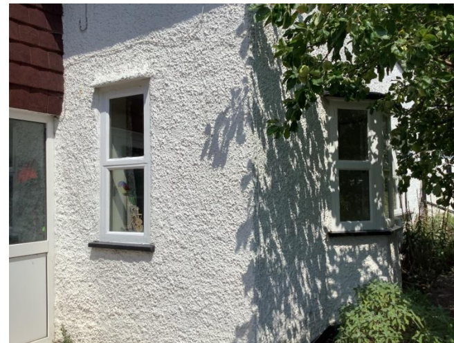
The 2 pane window on ground floor
