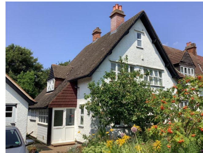
Angled front view of the house
