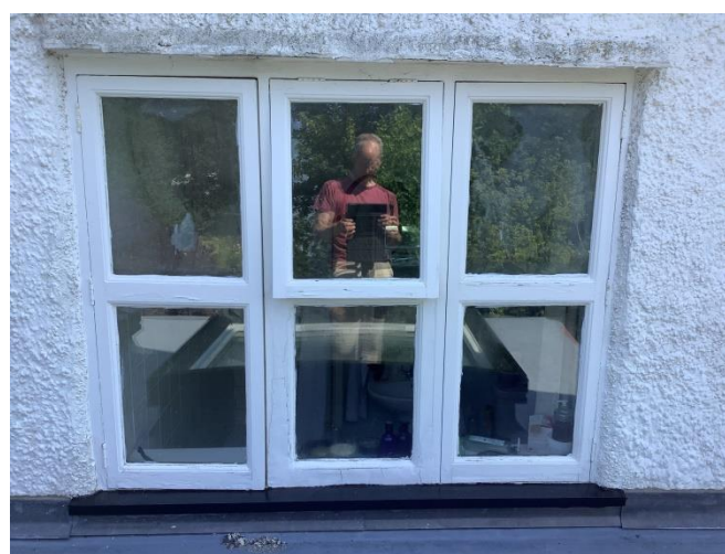
One of the two 6 pane windows on the rear of the house
