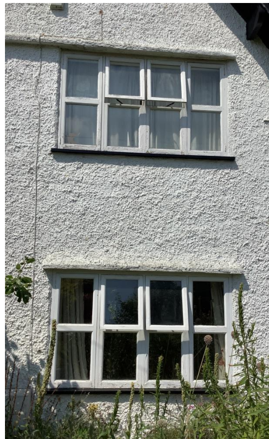
Two of the three 8 pane windows on the front of the house
