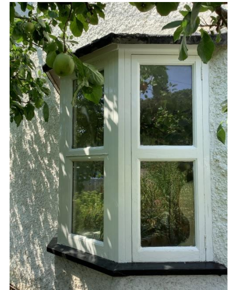
The 6 pane bay window on ground floor
