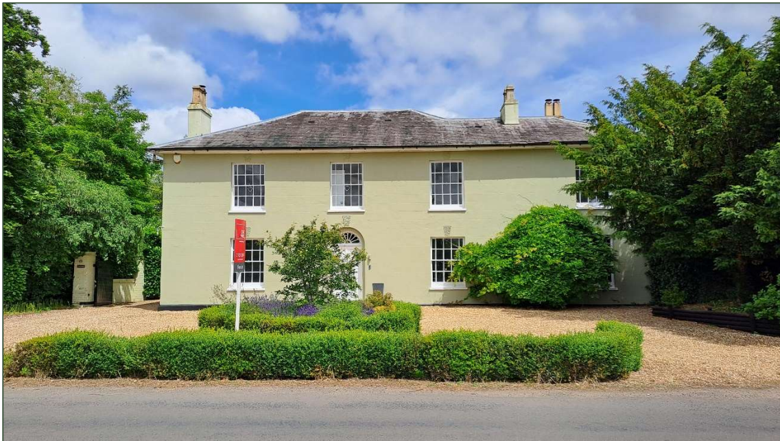
Plate 15: Beech House, facing Stevenage Road
