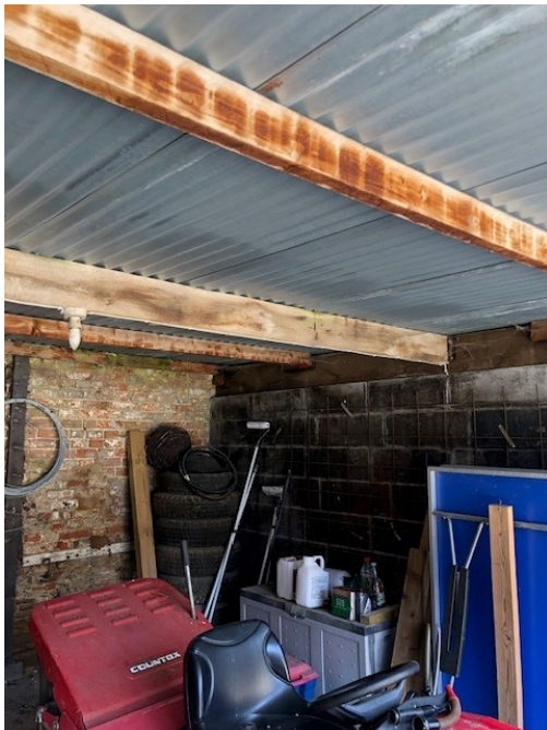
Photo – 8: Internal Blockwork Partition Wall
