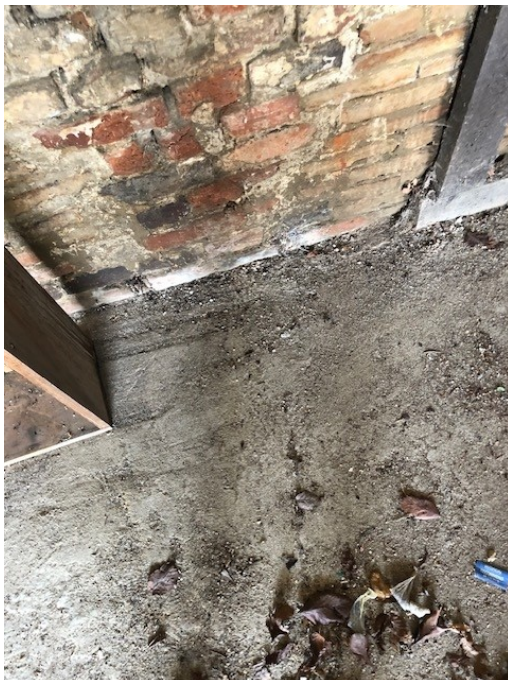
Photo – 7: Internal Concrete Slab
