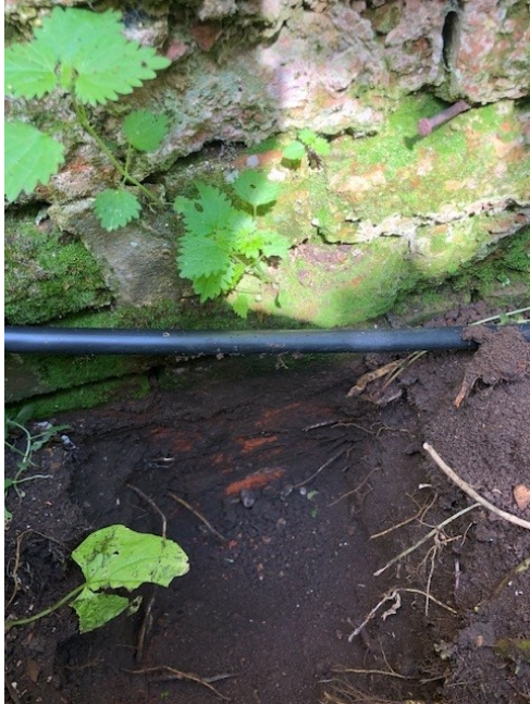
Photo – 6: Rear Wall Externally – Below Ground Level
