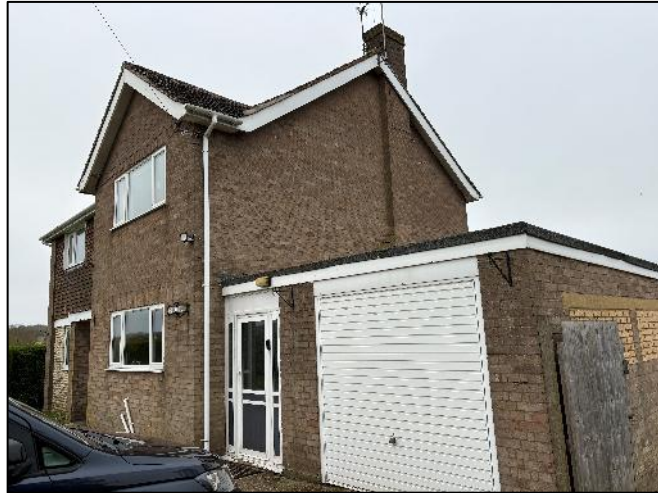
Photograph 1 North-eastern elevation of B1a and B1b
