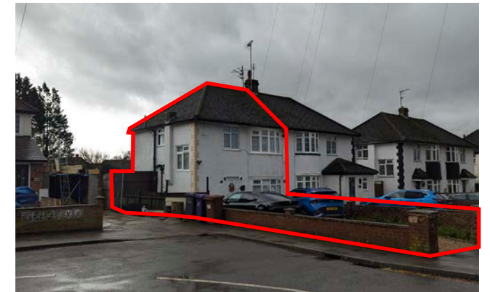
The Existing property viewed from Point A
